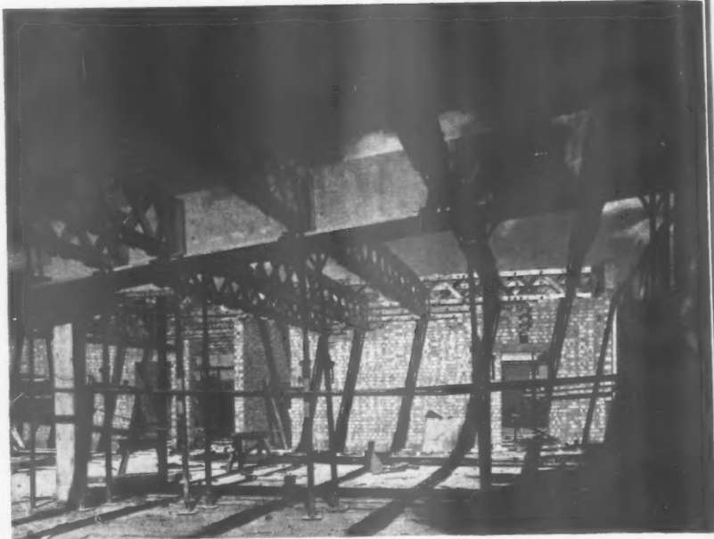
Trusses propped in position against in situ concrete beam, ready for end cleats to be bolted through beam.
