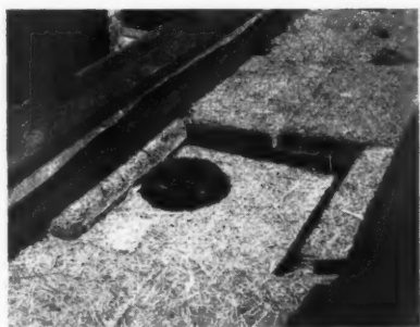
Above: partially completed clerestory roof. The hardwood windows are made in 12 ft. lengths and support the flat wood-wool roof over. See section on p. 206
