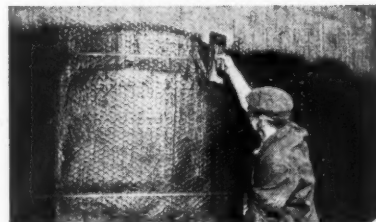
A variety of finishes can be applied to J & B Wire Netted Mattresses, Semi-rigid Felts, etc.
