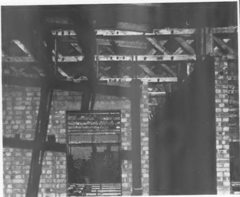
Junction between flat and sloping roofs. Honeycomb brickwork will be used for beam filling on top of the cross walls, to hold down m.s. cleats on the ends of trusses, and to allow ventilation between roof spaces.
