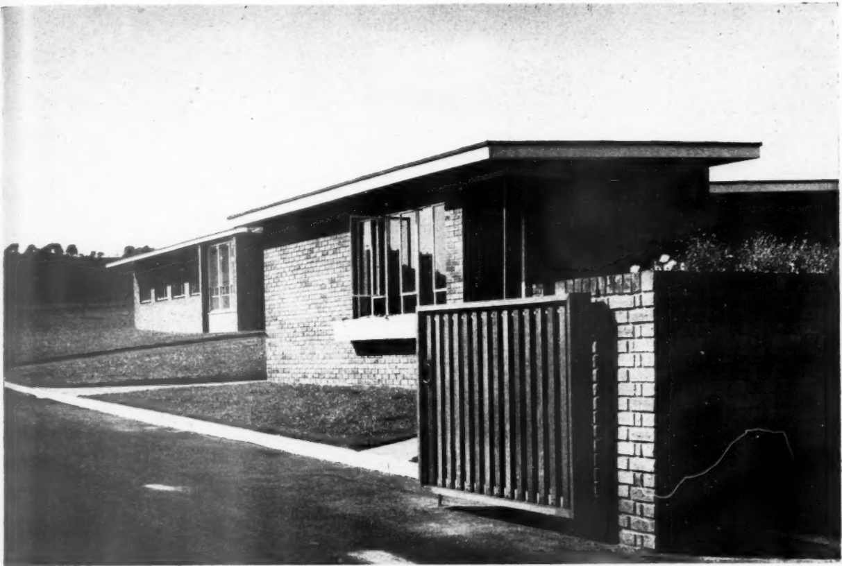
Above, the main entrance gates, south gatekeeper's office and the administrative offices in the background.
