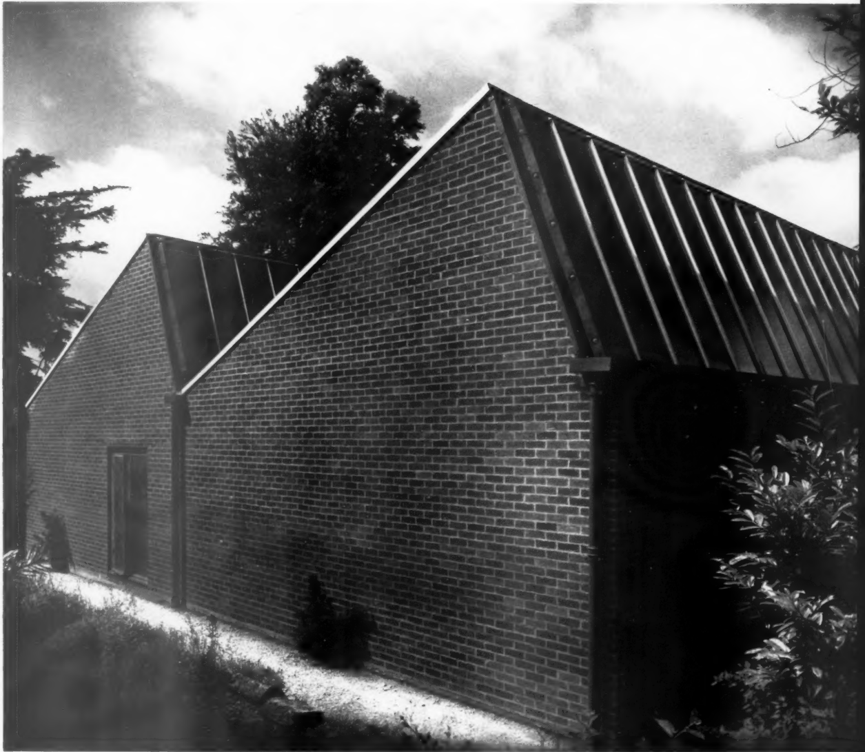
The glazing bars are of aluminium and the unglazed parts of the roof are covered with bituminous felt on reinforced wood-wool slabs.
