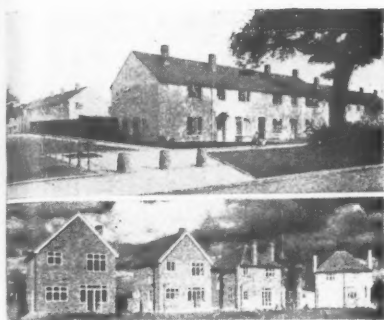
Top, what F. E. Ladly describes as "barracks," the Tile Hill Estate, Coventry, designed by City Architect D. E. E. Gibson—and, for comparison, a row of recently built villas.
