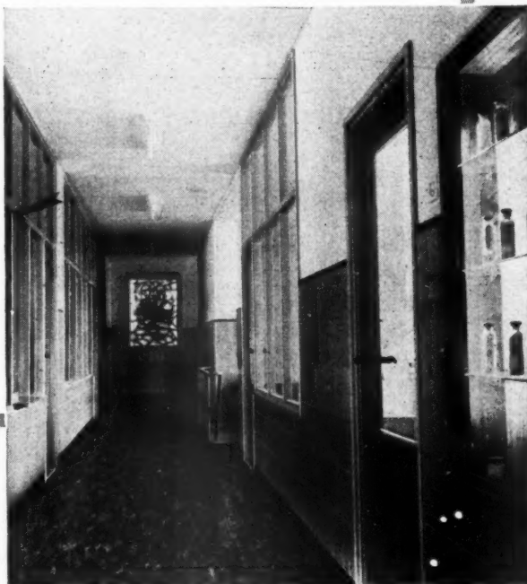
Entrance Hall, Doctor A. Verwey Chemical Laboratories, Coolhaven 32 — Rotterdam.
