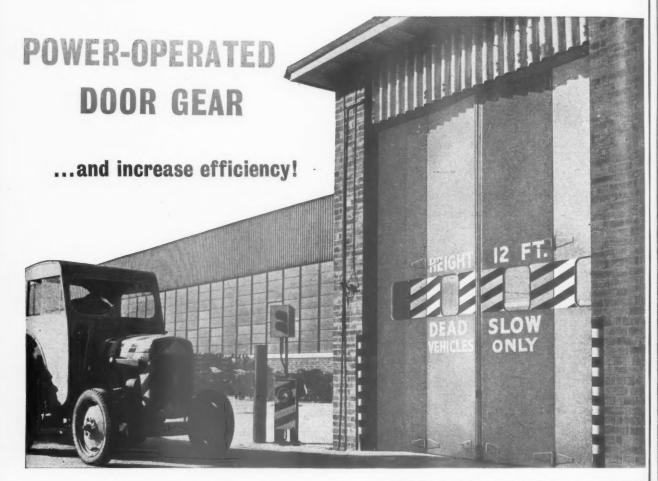
WHEN "DRIVE-IN" doors were required at Vauxhall Motors, Ltd., National Pneumatic-Peters' Automatic Door Equipment was specified. Photo-Electric Cell mechanism opens the doors when approaching traffic interrupts a light-beam . . . and they close automatically after a predetermined interval. Interlocking of two or more doors is also possible, permitting the operation of an air-lock or the retention of heat, humidity, etc.
