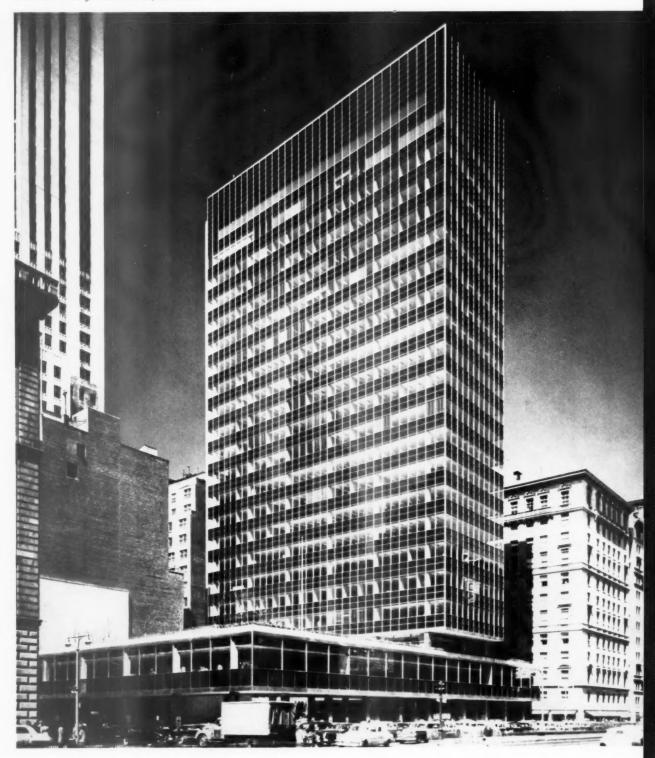
The mullions which are attached direct to the main supporting structure comprise two  $5\frac{1}{2}$  in.  $\times$   $1\frac{1}{2}$  in.  $\times$   $\frac{3}{16}$  in. steel channels which interlock but do not touch and thus serve as expansion joints. They are concealed on the outside by a coverstrip of 16 gauge stainless steel.
