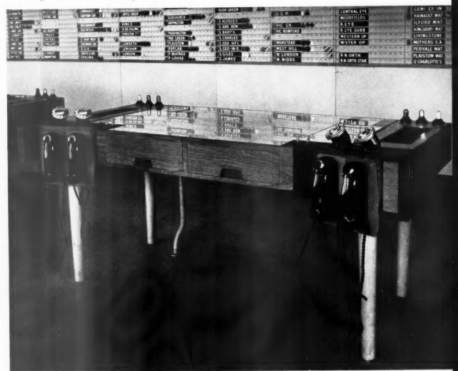
A handed telephone table for two operators for use in the Emergency Bed Service. The removable perspex top serves to cover a map of the London area to which the operators have frequently to refer. So that the top may be kept clear of obstructions the desk has been provided with filing baskets on either flank. The legs of the desk are screwed into fixing blocks attached to the underside of the blockboard sheet which forms the structural top of the desk.
