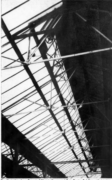
The illustration shows One set of Electrically operated Twin Tension Rod Gear with Counter-Balance Unit operating one continuous opening light, 74 $^{\prime}$ 0 $^{\prime\prime}$  long  $\times$ 5 $^{\prime}$ 0 $^{\prime\prime}$  deep. Note the Spiral Balance Wheel fitted at the end sprocket.
