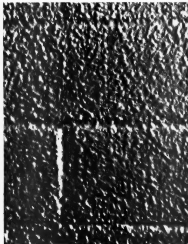
Stipple finish on flush-pointed brickwork
