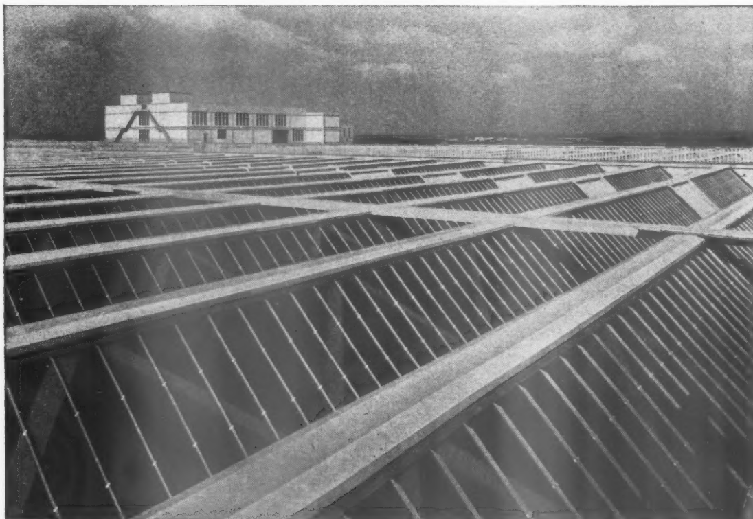
Part of the roof of the B.O.A.C. Headquarters at London Airport. The total area of glazing is approximately 280,000 square feet.
