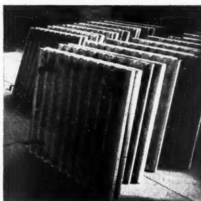
Top: manhandling an external partition unit. Centre: external partitions fixed and glazed. Bottom: precast vermiculite ceiling blocks stacked ready for fixing.
