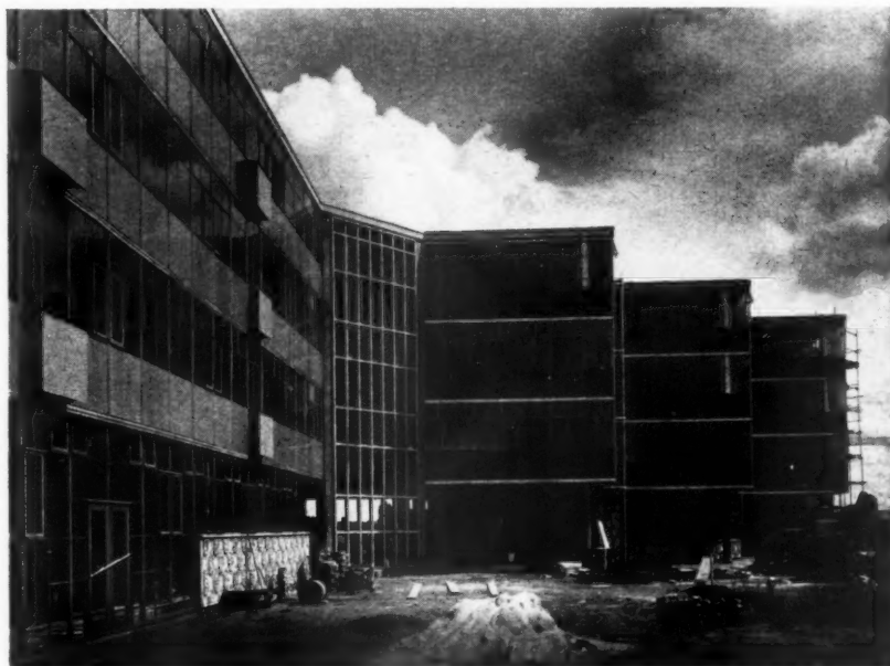
Above: general view looking towards the classroom wing. Note the projecting cases for the heating units on the left hand wall.
