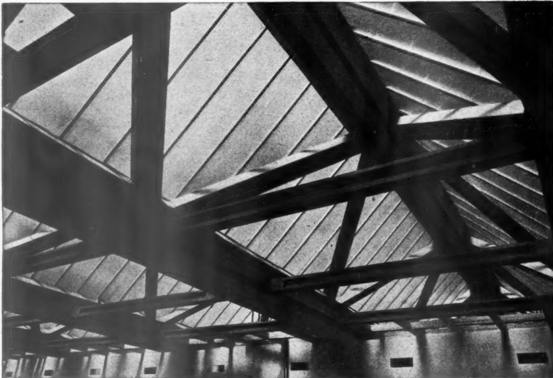
A close-up view showing the glazing and supporting structure from underneath.
