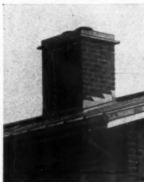
Flashing round chimney stack.
