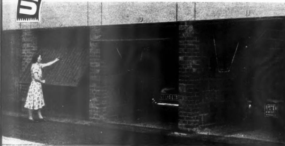
Top photograph (by courtesy of Messrs. G. S. Faulkner & Sons Ltd.) shows Model No. 1 fittings at The Reigate Garage Ltd. Model No. 1 is used when clearance over door is 16in. or more.
