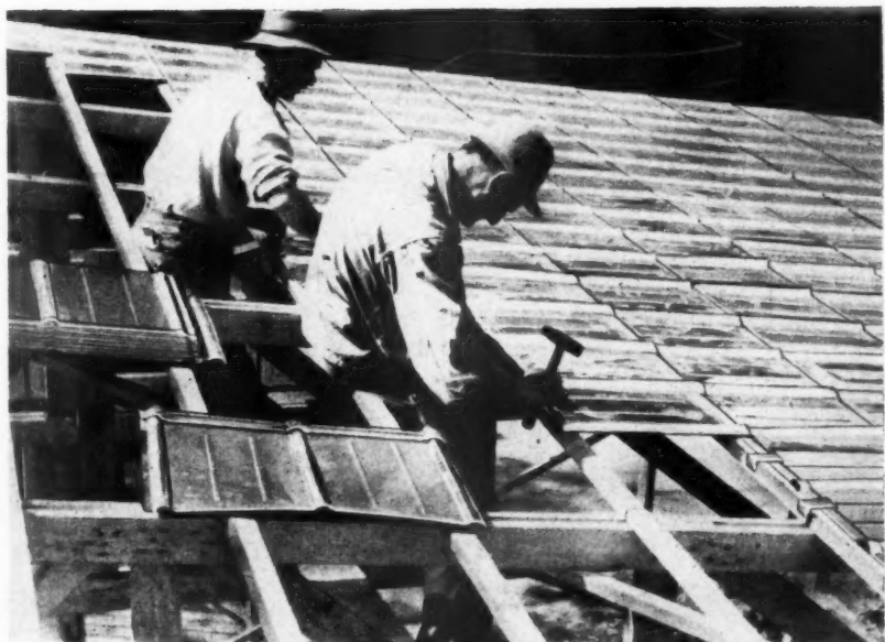
Fixing a Prefatiles roof.
