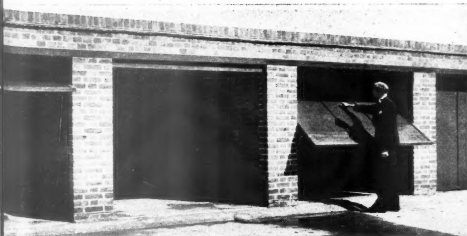
Lower photograph (by courtesy of Messrs. Rayners (Buildings) Ltd.) shows Model No. 2 fittings at a Guildford garage. Model No. 2 is used for clearances of 2in. or more.
