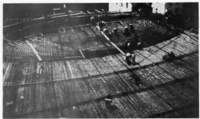
Hyperbolic paraboloid concrete shell roof at Karlsruhe. See note No. 19.181.
