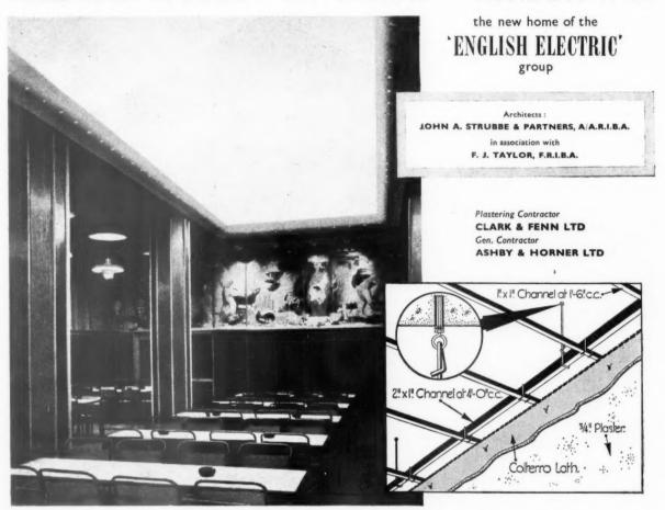
This attractive canteen ceiling, with a clean hygienic finish is suspended from the hollow tile floor. Contrasting acoustic and decorative treatments are used to advantage and COLTERRO Clay Lath ensures complete and permanent adhesion of the plaster.
