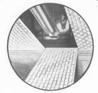
"DIFULITE" Cellular Sub-Ceiling combines modern, decorative treatment with overhead lighting (over the complete ceiling if required) soft, diffused and comparable with daylight, and is ideal for concealing unsightly structures, without costly alterations.
