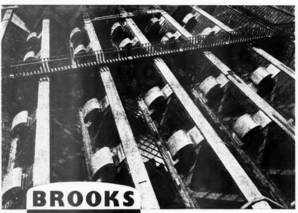
The installation of twenty 36" 'Brooks' Fan Powered Special Roof Extract Units at London Airport.
