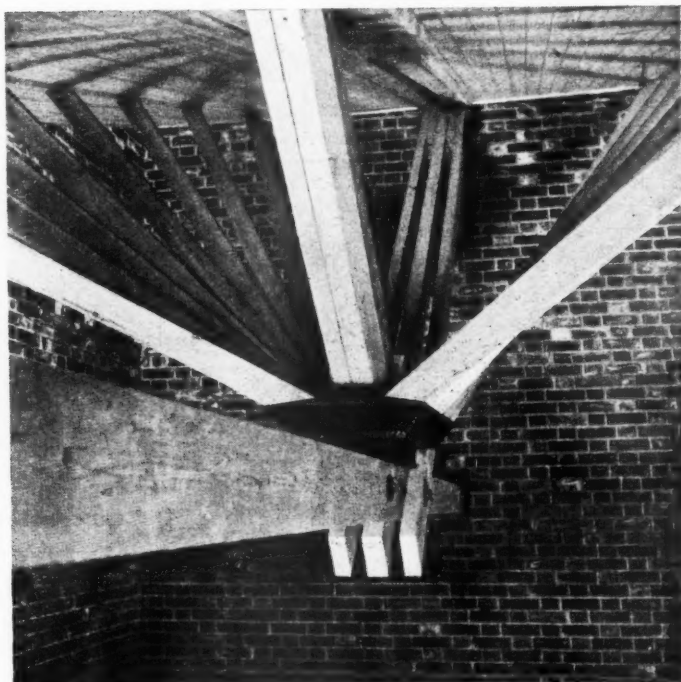
Top, plan of a concealed window designed to throw light on the speaker's platform in Alvar Aalto's Town Hall at Saynatsalo. Above, the baffled window. Right, part of one of the two unusual timber trusses spanning the town hall. These illustrations are from a book on Alvar Aalto reviewed by ASTRAGAL this week.
