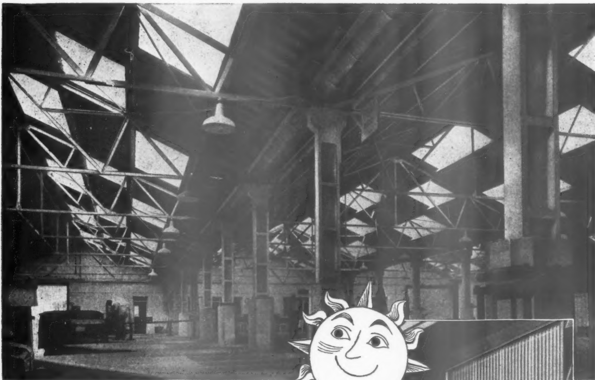
Corrugated 'Perspex' gives excellent day-lighting at the East Sussex Growers Ltd. packing station at Polegate, Nr. Eastbourne, Sussex.
