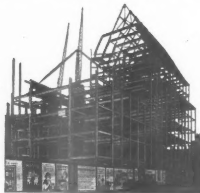
A view of the skeleton framework during construction.
