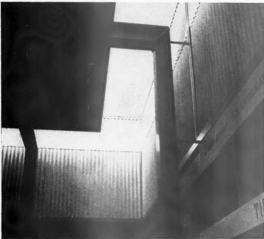
Above, a detail of the construction of the concourse of Vällingby Station on the Stockholm underground, showing welded steelwork and simple asbestos panelling. Below, tiled columns and a tiled floor in the Kungsgatan Station and, right, part of the Blackeberg Station concourse.
