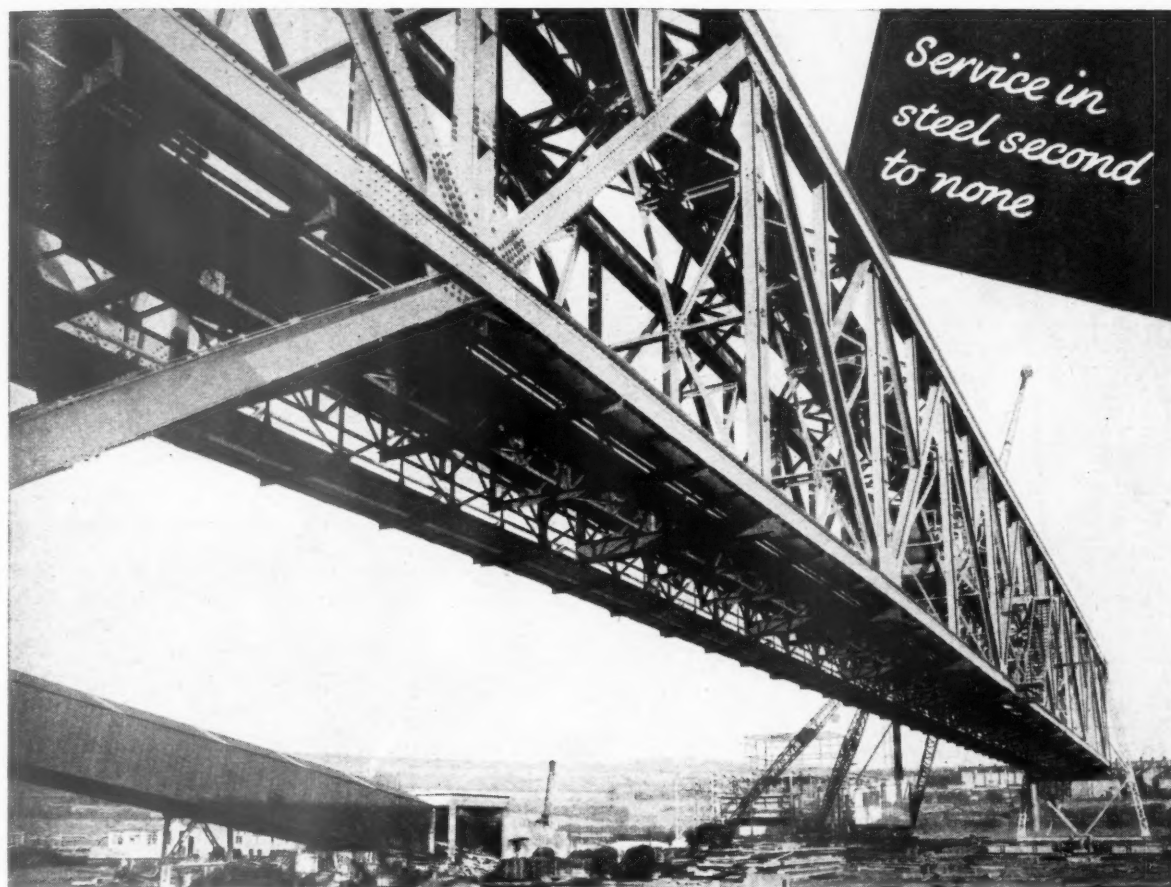
Structure for 300 ft. Span Transporter Crane. Manufactured to the order of Mitchell Engineering Co.
