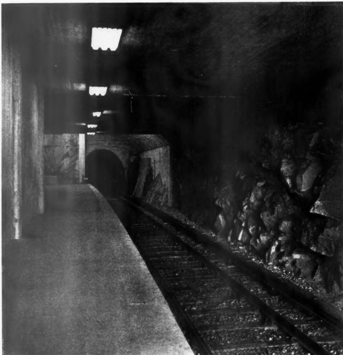
Above, Vällingby Station on the new Stockholm underground railway, showing the concrete left untreated from the shattering and the rough, blasted, granite walls which contrast so favourably with the glass, aluminium and grey plastic panels of the surface buildings, left.
