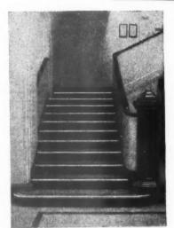
Don Plastic-filled Stairtreads in use on the staircase of a Government Department The ribbed surface of the plastic
