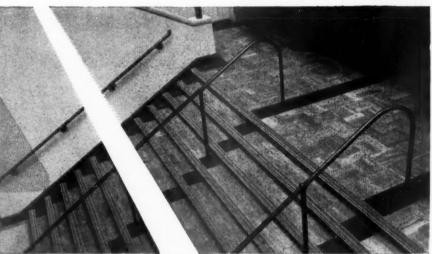
However much the patrons of the Ayr Ice Rink slip and slide on the ice, they are sure of a firm foothold on the entrance stairs. For the owners have taken the wise precaution of fitting double channelled Ferodo Stairtreads. Protective aluminium nosings outline each step; two wide treads of attractive but tough, red composition, give a firm, confident grip to the wettest shoe . . . safely speed the feet of the most impatient youngster.
