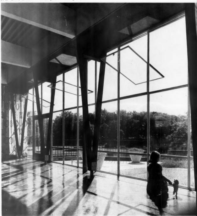
The form of the stanchion is chiefly determined by the need to provide a connection with the beams strong enough to overcome wind pressure. The timber used is red meranti. One plywood gusset plate is glued to the stanchion in the shop and the other is glued on the site after fitting the beam in position.
