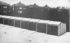
'Alborough' prefabricated concrete units, when treated with Alkali Resistant Chlorinated Rubber Paint, are equal in appearance to traditional timber construction.
