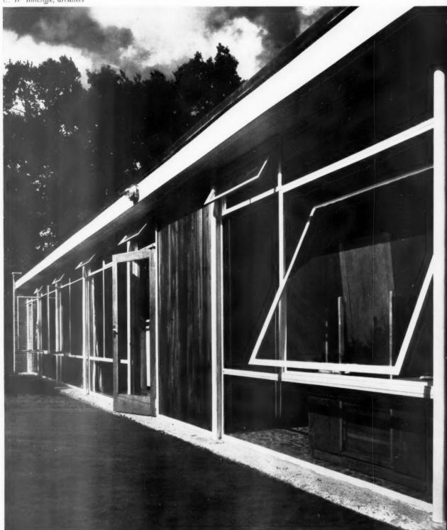
The windows are fabricated of medium universal sections, hot-dip galranised with spring steel metal beads. The columns, which are of 23 in. hollow steel tube with welded caps and bases, are 1 in. clear of the mullions to ullow for painting.
