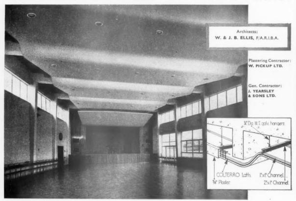
Complete freedom of design is possible with the COLTERRO Lath system of suspended ceiling construction. Any profile can be faithfully interpreted, and irrespective of shape a perfect key for the plaster is always assured.
