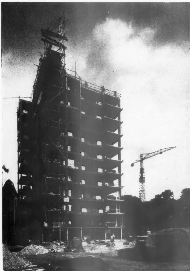
Fig. 1. General view of block from ground level showing staging for hoist.
