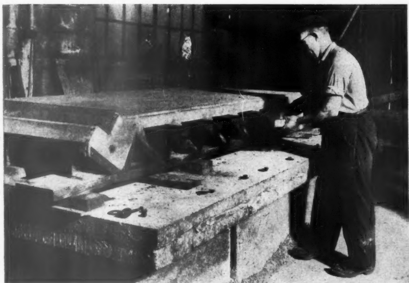
Fig. 10 (above). Withdrawing cores from a precast stair flight. Fig. 11 (above right). Hoisting a precast stair into position. Fig. 12 (right). Raising a balcony off a shutter. Fig. 13 (extreme right). Lowering an edge beam into position. Note temporary safety rail.
