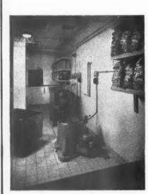
The laundry, which is described in detail on page 278, has a floor of buff quarry tiles and white walls. In the foreground is the hydro-extractor, with the washing machine behind it. In the far wall are the issue and return hatches for towels. Hot and cold water is supplied to the washing machine: this is found more economical than the raising of heat by the electric coil in the machine.
