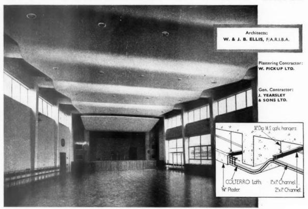
Complete freedom of design is possible with the COLTERRO Lath system of suspended ceiling construction. Any profile can be faithfully interpreted, and irrespective of shape a perfect key for the plaster is always assured. The arresting ceiling illustrated provides the correct acoustic treatment for the Assembly Hall and a clean, light reflective surface. This is one of the many school contracts entrusted to us throughout the country.
