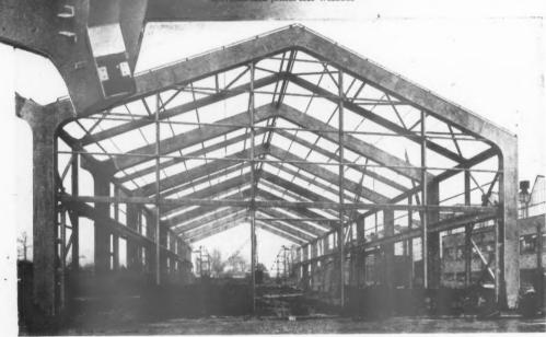
Main Building: 338 ft. long, 80 ft. span. Transverse Building: 80 ft. long, 64 ft. span.
