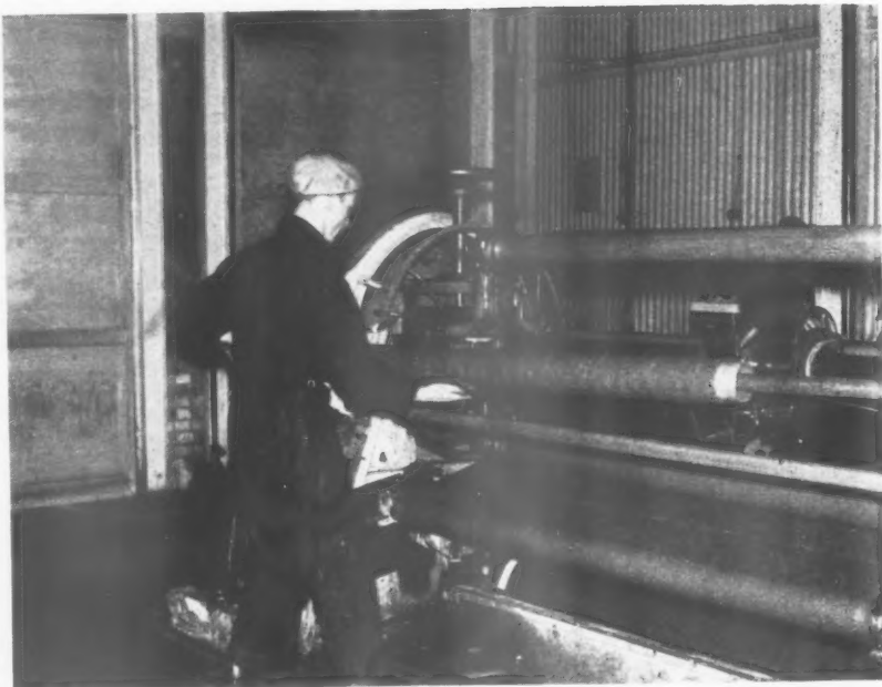
Fig. 1. The pulp stock is pumped to the pipe-forming machine where the fibres are deposited on to a mandrel in layers and formed into a pipe of constant thickness.
