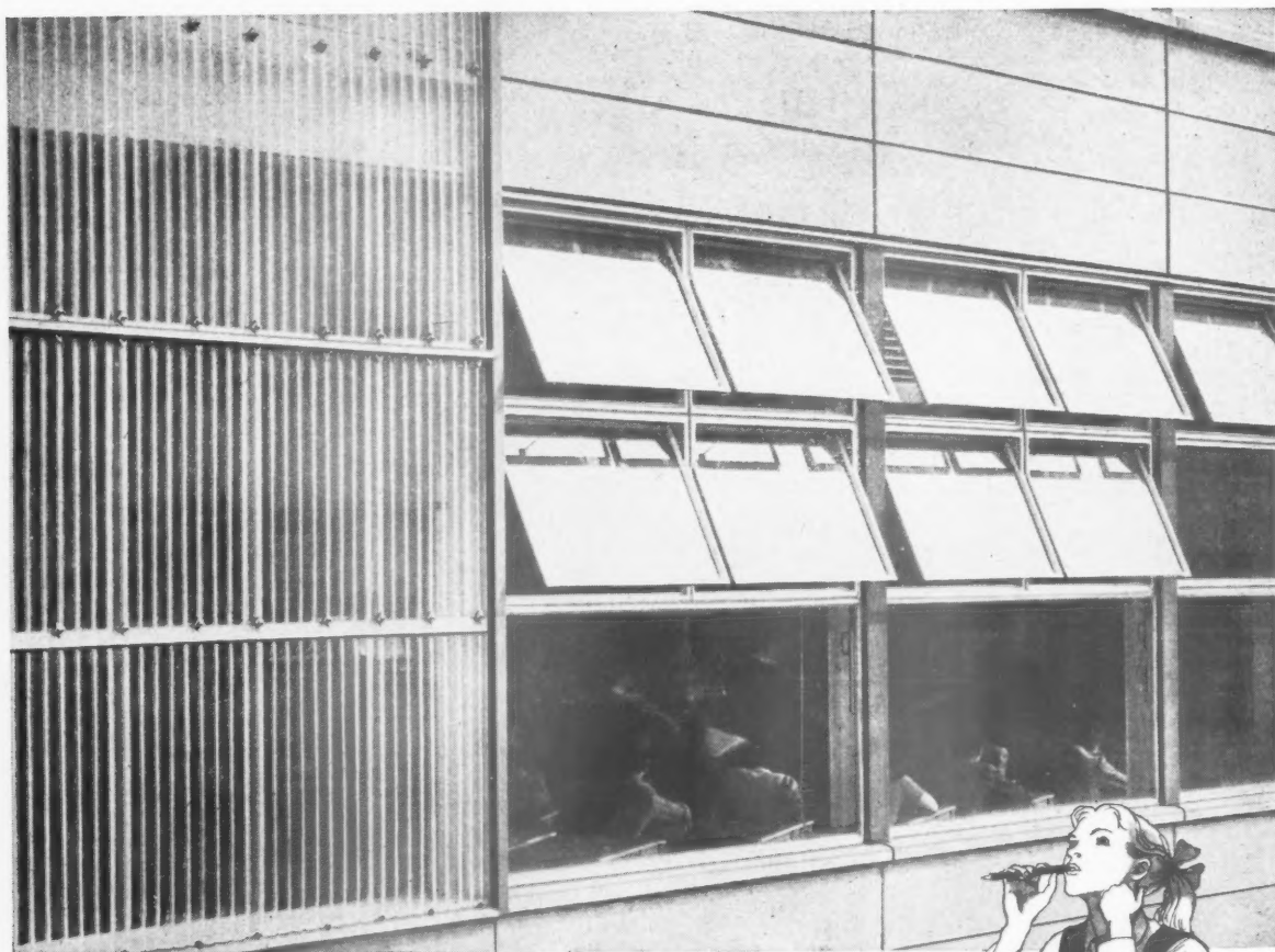
Corrugated 'Perspex' used vertically over two stories at The Barclay School, Stevenage, Herts.
