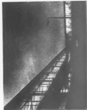
The top photograph shows the north-east corner of the office block and, in the foreground, a single-storey block, which contains part of the photographic department. Nearly all the external walling is non-load bearing. The aluminium glazing on the first floor oversails 1 ft. 8 in. beyond the column grid. The glass panels under the first
