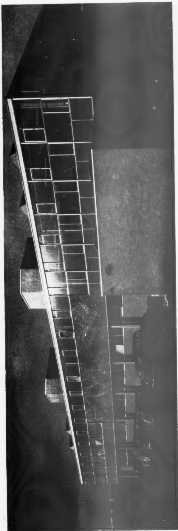
The top photograph shows the north-east corner of the office block and, in the foreground, a single-storey block, which contains part of the photographic department. Nearly all the external walling is non-load bearing. The aluminium glazing on the first floor oversails 1 ft. 8 in. beyond the column grid. The glass panels under the first
