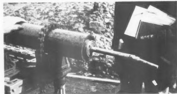
Fig. 2 (top). Cutting a 4-in. pipe with a saw.
