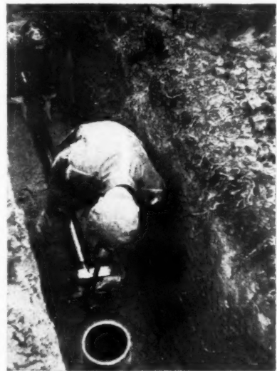
Fig. 7 (above). The joint is driven up on a block of wood placed across the last sleeve. Note: The 2 ft. 6 in. trench is more than wide enough. Fig. 8 (below). Backfilling in sections to hold pipe in place. Note: Laying in very wet conditions. Fig. 9 (bottom). Pitch-fibre oblique junction 4 in. to 6 in.
