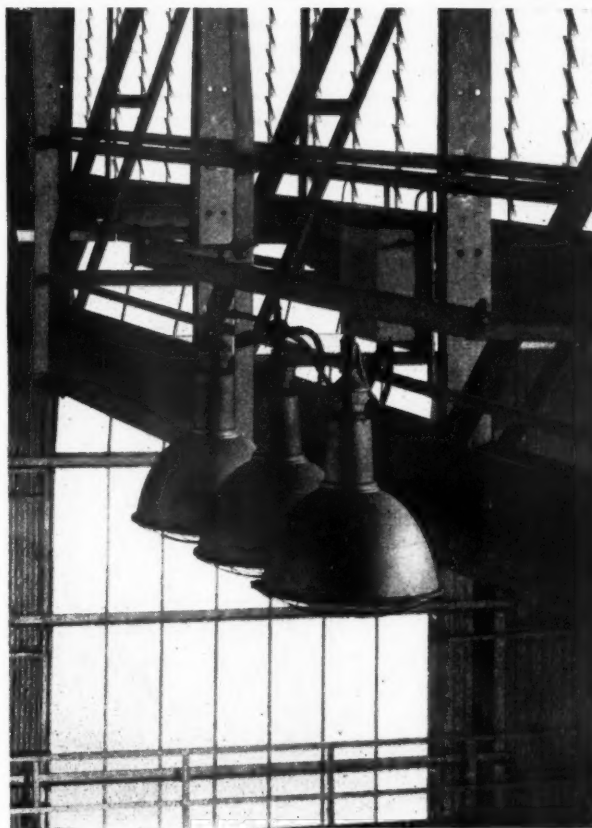
Fig. 6, above, high bay lighting with 1,000 watt mercury vapour (MA/V) lamps spaced at wide intervals in a steelworks. Fig. 7, right, "blended light" installation in a steelworks showing control gear and walkway for maintenance.
