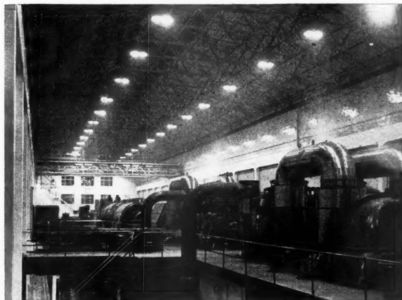
Fig. 5, a "blended light" installation—i.e. mercury discharge lamps and tungsten filament lamps used together—in a turbo-alternator hall.
