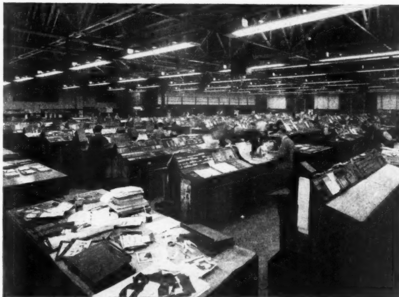
Fig. 3, above, low bay lighting with hot cathode fluorescent lamps mounted on continuous trunking system. Fig. 4, below, cold cathode industrial lighting installation in a printing works—low bay lighting.
