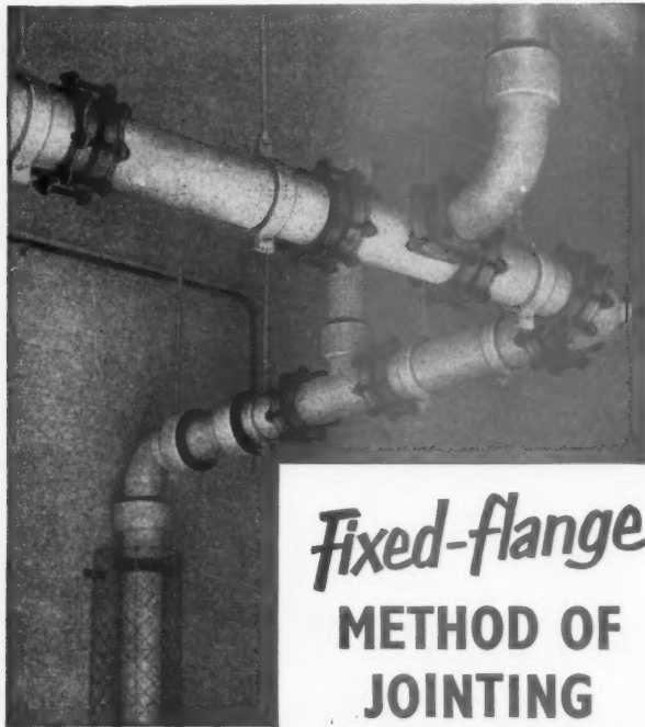
Royal Doulton acid proof white chemical stoneware pipe lines at the Imperial College of Science & Technology, South Kensington, showing the fixed flange method of jointing.
