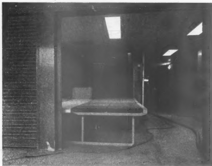
The starting point for one of the luggage conveyor belts on the north west, or landside, of the building. The control box and telephone is above and to the right of the belt.
