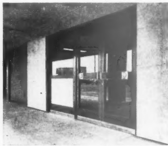
Typical entrance doors (viewpoint C) to one of the passenger channels. The doors are of hardwood with metal trims. On the left are the vertical-sliding steel shutters which give access to the conveyor-belt for the luggage of passengers using this channel. The walls are dressed with artificial stone slabs.
