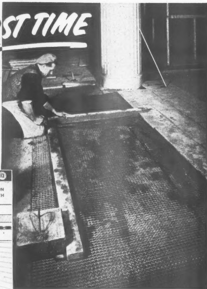
QUIL-LATH Flooring being laid at Messrs. Lewis's, Ranelagh St., Liverpool
