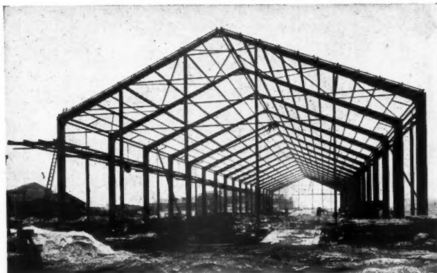
Welded Transit Shed for British Transport Commission.
