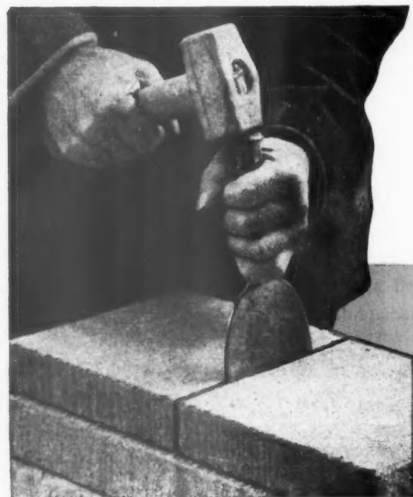
Cutting Thermalite blocks with a bolster
