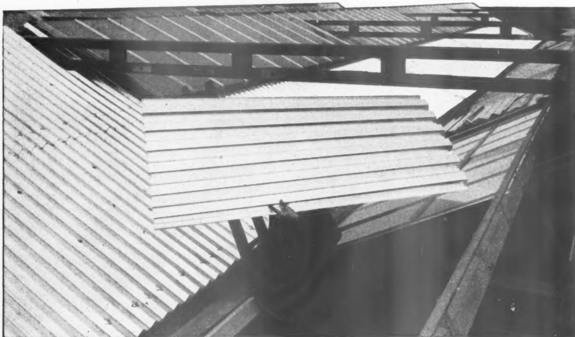
A roof at the Huddersfield works of Messrs. W. H. Heywood & Co. Ltd., being covered with Noral 'Industrial' sheet.
