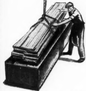
Cold-bath method of applying pentachlorophenol.
