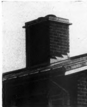
Flashing round chimney stack.
