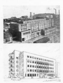
cladding, glass blocks used extensively to avoid corrosion. Assistant, A. E. Wintle. Sketch of new offices at Westgate, Leeds, now under construction. Steel frame, green Westmorland slate cladding, Cornish granite, Portland stone and quartzite. Right, offices for the Yorkshire Ouse River Board, Leeds, exterior, and the board room. Assistants: W. H. Crocker, Kenneth Warman.
