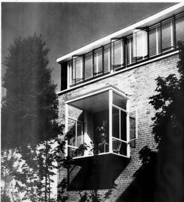
The bay window has been built into an existing brick-faced stone wall and is supported on a framework composed of three lengths of 4-in. by 2-in. ms channel. This framework, which is mitred and welded at the joints, is bolted down to a concrete sub-floor inside the building and, outside, provides the forward edge to the bay. The glazing in the lay front is in the form of a fixed light in 4-in. polished plate glass to give the maximum unobstructed view from the room behind.
