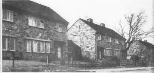
concrete roof to classrooms, woodwool slabs on steel trusses for halls. A church with parish hall, at Seacroft, Leeds. This page, a terrace of three houses at Linton, left, and five pairs at North Rigton. The former cost £1,737 per house. The internal area is 1,008 sq. ft. The latter cost £1,547 per house for z floor area of 1,037 sq. ft. Both are constructed of old stone
