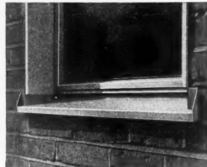
Zinc weathering on window sill.
