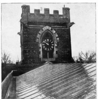
Super Purity Aluminium is a plumber's metal; 99.99% pure and the most ductile and workable form of aluminium obtainable. It is a permanent roofing material which costs considerably less than the more traditional plumber's metals, although it is capable of lasting just as long. Super Purity is particularly adaptable to church roofs both from the economical and the practical point of view.
