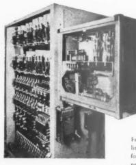
The main lift controller and electronic control equipment, which can be sited in any convenient position. Right: Factual speed/time curves for this electronically controlled lift Below: Drum mechanism, embodying campand followers of the control gear, photographed across the lift shaft.
