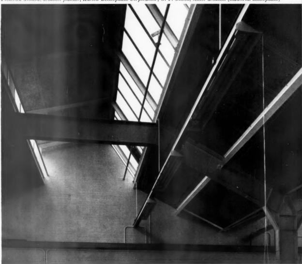
The sloping glazed surface faces towards the north. Heating pipes run at the foot of each line of glazing to prevent downdraughts onto the floor space below.
