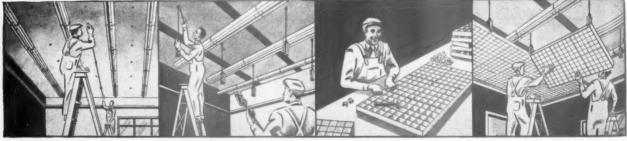
Measure off ceiling and locate hanger positions.
