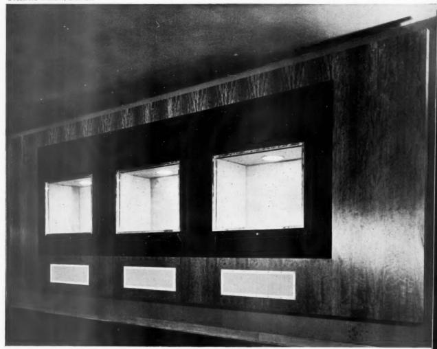
The window fronts are openable. They are top-hung and ride on a pair of quadrants which slide between the sides of the showcases and the intervening brick piers. They are secured by a mortice cupboard lock, the escutcheon of which can be seen projecting through the surround. This surround is covered with full-grained cowhide, dyed dark blue. The main panel is veneered in figured teak.
