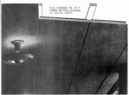
Typical Installation of "Supacoust" Tiles
