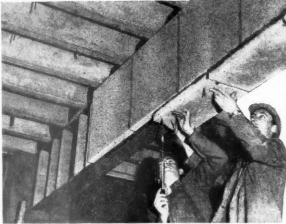
Meta Mica sectional cladding being fitted to structural steelwork at a large store in Coventry
