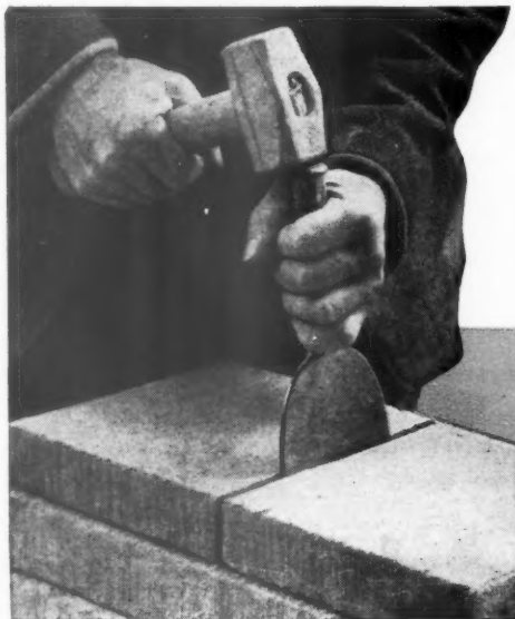
Cutting Thermalite blocks with a bolster
