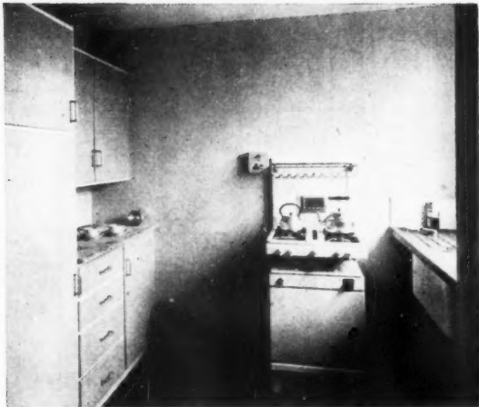
Above: a typical kitchen. Standard wood dresser units, broom cupboard, double draining boards, and a ventilated larder are provided to each kitchen. Walls are cream (7.5 Y 9/6), doors and doors to units pale blue (7.5BG 6/2), frames to fittings blue/white (5.0 B 9/2) and ceilings white. Above right: where the first floor projects over the ground floor the under-side of the precast, prestressed beams and the 3-in. solid concrete pots are exposed and simply painted.
