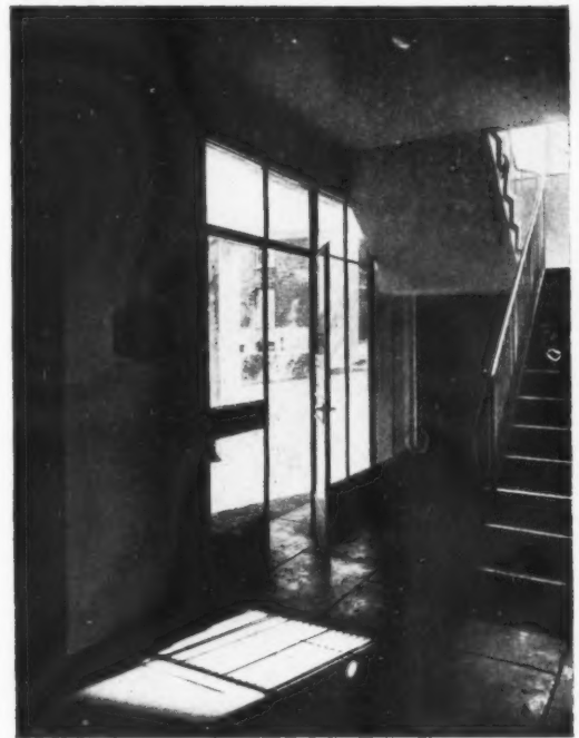
The entrance lobbies at ground floor level are paved with 3-ft. by 2-ft. precast concrete slabs laid breaking joint on a damp-proof membrane. The steel entrance doors are glazed in georgian wired glass.
