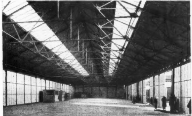
Storage Shed, Quayside, Newcastle-on-Tyne
