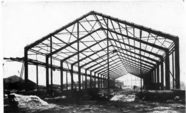
Welded Transit Shed for British Transport Commission.
