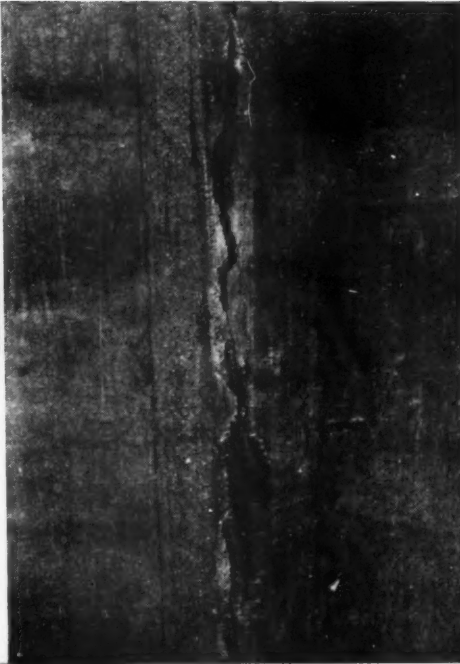
On the Silcock Silo, steel reinforcement had corroded and disintegration of the concrete was taking place, as shown in the first illustration on the right. At the extreme right the same detail appears after Pyrok was used for protective and decorative treatment. Work was executed by C & T (Pyrok Contracts) Ltd. London
