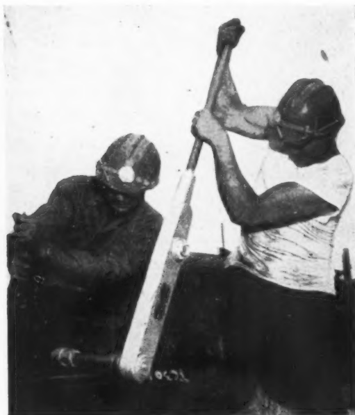
Fig. 2. (above). Method of fixing showing, left, the bolt head held by a hand wrench and right, the nut being turned by a pneumatic impact wrench. Fig. 3. (right). Checking high tensile bolt with a torque wrench.
