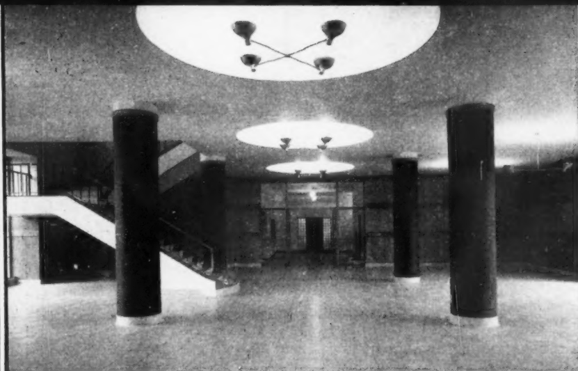
Entrance Hall, heated entirely by panel coils embedded in the false ceiling.
