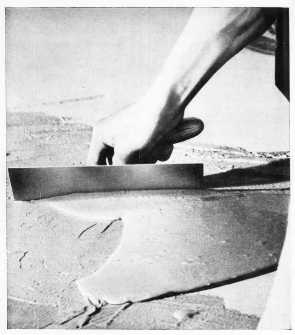
Picture of a Catesbys craftsman laying lino That is the adhesive he is spreading. Knowing the right adhessive for a particular sub-floor and having the men to apply it correctly is the most important single thing in perfect lino laying.
