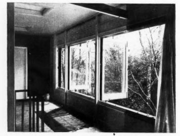
Landing on first floor overlooking garden to the south. Softwood T & G boarded floor on timber joists to receive linoleum at later date. Skim coated plaster board panels occur above and below the window line and form the ceiling. Colour: Return wall at the end of the landing, red 7 5R 14/6 (Munsell Range). All other exposed surfaces, broken white with the exception of the stained and cellulosed stair.
