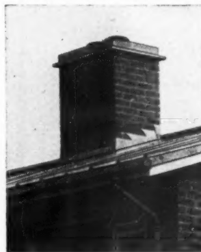
Flashing round chimney stack.
