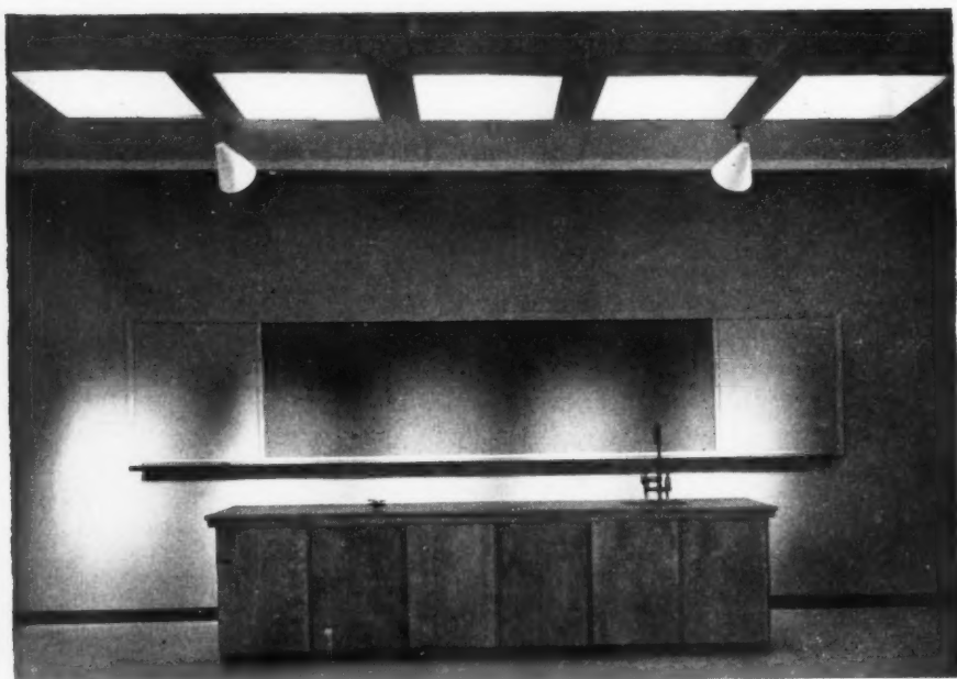
Top: one of the laboratories in the science block showing the fitted furniture designed for the school; to the left of the blackboard is a fume cupboard. The cupboards are pre-made and the tops were cut to fit on site; both are in Yugoslav beech. Above: a demonstration bench complete with chalkboard, pin-up and both direct artificial and natural roof lighting. Left: a new self-trapped dilution pot which was designed for the school and is incorporated in the bench tops.
