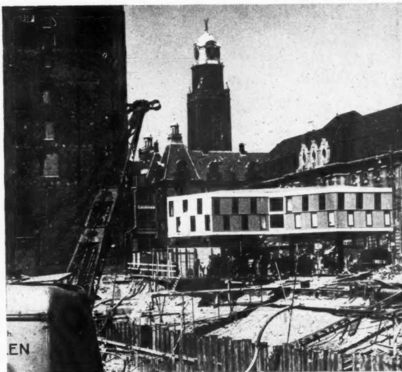
In recent years there has been a slow but steady improvement in the standard of site-huts. Even so, few come up to the standard of this hut on a building site in Rotterdam, a picture of which Rachel Caro has sent to ASTRAGAL. Painted in white, blue and red, with fluted asbestos panels, it stands on three columns, thus keeping the ground on this confined site as free as possible from obstacles.
