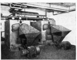
Riley Robot Stokers firing central heating boilers at a York school.
