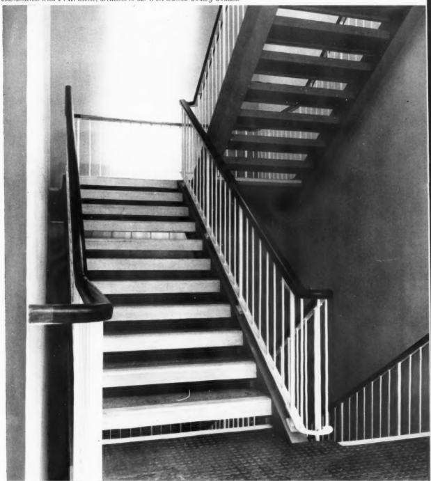
The precast concrete treads are supported on projecting shelves formed in the post-tensioned string beams. The welded m.s. balustrade, which runs both sides of the stair, is supported on tube uprights grouted into pre-formed sockets in the string beam.
