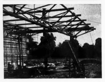
core of the edge beam which is, in effect, a lattice beam, made from two sets of 3-in. × 2-in. angles boilted to the hanger ends and forming the top and bottom members of the beam. The hangers along the short ends of the high level roof are welded to angles which are bolted to the endmost channels. The surrounding low level roof trusses and beams are supported from the edge beam. The low level bays are 8 or 9 ft. wide, and are all horizontally cross-braced with 2-in. × ½-in. mild steel flats.
