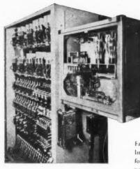
The main lift controller and electronic control equipment, which can be sited in any convenient position. Right: Factual speed/time curves for this electronically controlled life Below: Drum mechanism, embodying cams and followers of the control gear, photo-graphed across the lift shaft.
