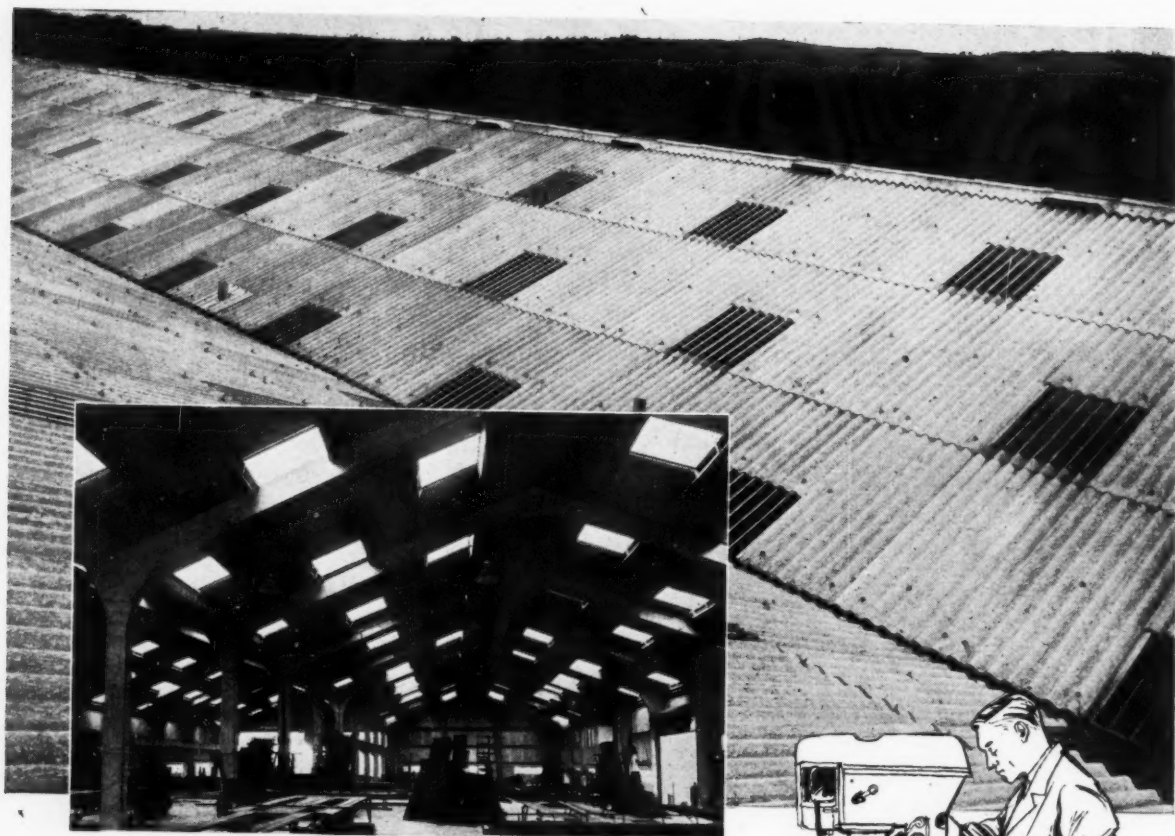
Corrugated 'Perspex' roof lights in the new factory of The Square Grip Reinforcement Company (Bristol) Ltd. The architect is A. E. Powell, A.R.I.B.A., A.I.Struct. Eng.. Roofing—W. R. Davey & Sons.
