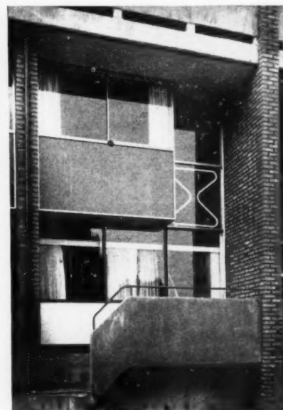
The first flat in the City of London's Golden Lane Housing Scheme has been completed and above left we show the living-room, with its cantilevered pre-cast concrete staircase on the right, and the kitchen hatch beyond. Above right is part of the facade; the panels below the aluminium sliding windows are painted blue. The architects were Chamberlin, Powell and Bonn.
