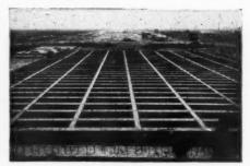
3 Part of Deck Supporting Structure prior to erection of Steel Plating. Approx. 730 tons of steelwork were used in this contract.
