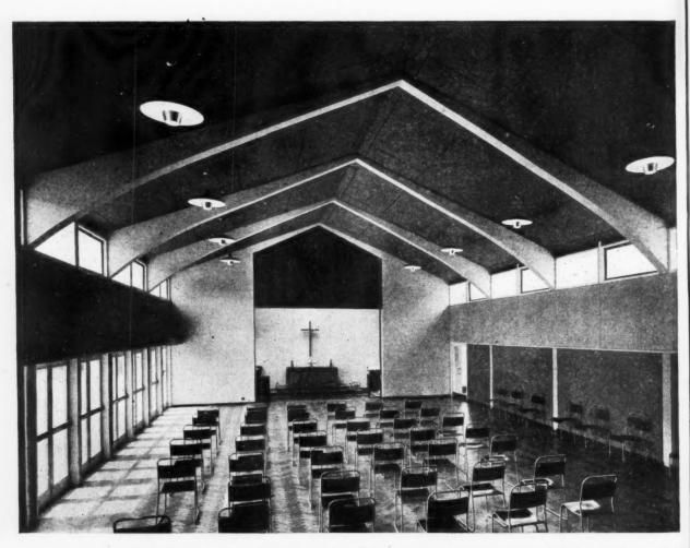
A general view from the stage end of the hall. The floor is wood block laid in herringbone pattern and wax polished. The horizontal strip above the row of double doors on the left is in  $\frac{1}{16}$ -in. fibreboard nailed to 3-in. by 2-in. s.w. studding. The dark panels behind the chairs on the right are  $\frac{2}{8}$ -in. plastered breeze blocks with a strip of  $\frac{1}{16}$ -in. fibreboard above nailed to battens. The flanking walls to the chancel are in
