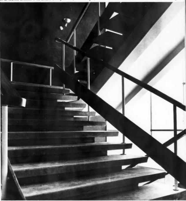
The two rolled steel channels forming the strings of this staircase are encased, for fire protection, in vermiculite rendering sprayed on expanded metal. Treads and risers were precast but the landings were formed in-situ.
