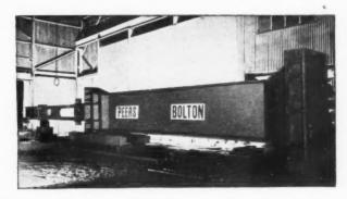
One of 16 all-welded stanchions each weighing 21 tons.
