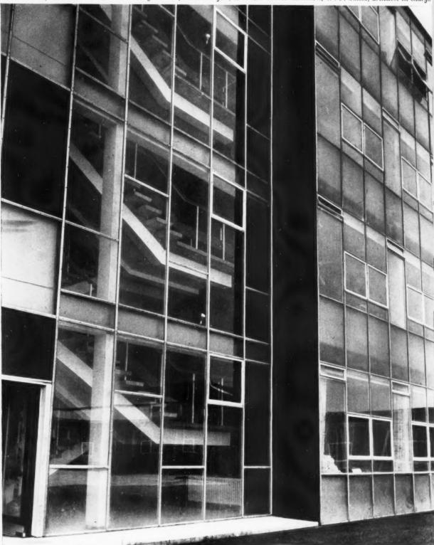
This glass curtain walling is formed of mild steel mullions and transoms of cruciform section, supported at each floor on a horizontal m.s. angle fixed to a strap welded to the beam.
