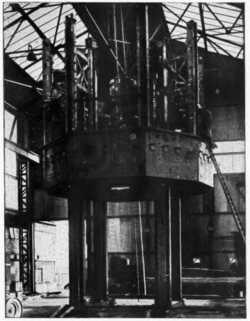
Framework for the new heavy water moderated reactor E.443 which is being built at Harwell. The structure has been fabricated by us for Messrs. Head Wrightson Processes Ltd.
