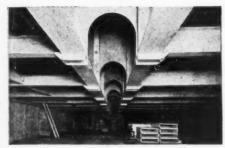
1 View of 70-ft. long Twin Welded Girders underneath Arrested Landing Deck.
