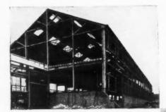
Heavy steel framed structure from design to fabrication and erection, 160 tons erected in 2 weeks.
