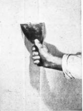
Final coat of GYPROC Joint Filler applied with a 5" wide rigid joint filling knife.
