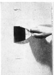
Apply a thin layer of GYPROC Joint Filler into recess with a 4" wide flexible joint filling knife.
