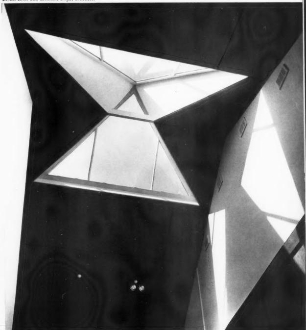
A lantern light with glazing at 45° has been contrived over the ridge of a 2210 pitched roof. The ridge board of the roof penetrates the framing of the lantern and is visible from below. The lantern is sheathed in superpurity aluminium to match the patented "clip-on" type aluminium covering used on the main roof. The object of the designers was to obtain a structure which, while giving a large glass area, would be light in weight but very strong.
