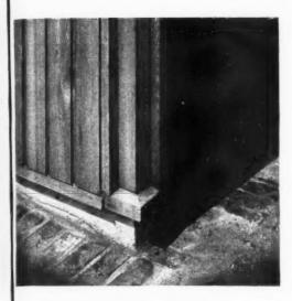
Left: the external corner junction between a solid panel and a window panel is formed with a corner plate and post (see detail drawing on page 331).
