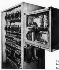
The main lift controller and electronic control equipment, which can be sited in any convenient position. Right: Factual speed/time curves for this electronically controlled lift Below: Drum mechanism, embodying cams and followers of the control gear, photographed across the lift shaft.
