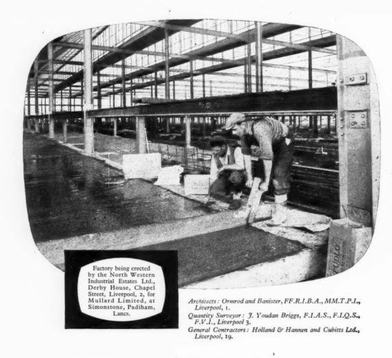
The Basement Floor was laid in alternate rectangular panels between the foundation beams approximately 12' 0" wide, and the concrete composed 4:2:1 6" thick, waterproofed by the addition of 5 lbs. of 'PUDLO' Brand Powder to each 100 lbs. of cement.
