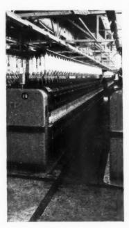
Above: the mill floor slab has been laid in bays of 38 ft. by 20 ft., with joints between adjoining bays, dimensions having been determined by the sizes of the spinning machines. There is a 1-in. granolithic floor finish, and joints are masked by 6-in. × 3-in. × ½-in. rebated quarry tiles, set in mastic.
