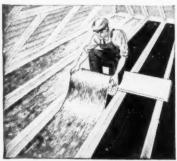
will reduce the loss of heat through a roof-area by at least 70%. This loss, in the average house, is about one-third of all the heat lost in various ways from the structure as a whole.
