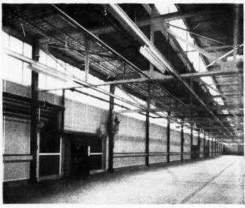
Above left, the 8 in. by 6 in. by 35 lb. R.S.J. side columns take up any movement on steel roller bearings. The rollers are in a grease-packed box, the top of which is level with the finished floor level. Details above floor level are similar to those already described for the central columns. For detail drawings of these columns see page 363.
