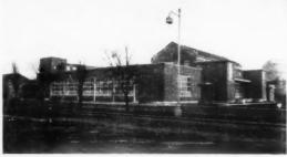
1949. To save steel, which was in short supply at the time, load-bearing walls with centre columns were used. The block accommodates 60 technical officers and 200 laboratory assistants. Floors are of precast concrete hollow beam construction with approximately 7-in. of foam slag screeding to cover ducts and floor drainage channels. Heating and ventilating is by a modified plenum system. Cost: £135,000, or 55.  $2\frac{1}{2}J$ . per ft. cube.
