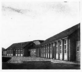
a county school for 240 at West Hartlepool. The assembly hall acts as a dining room. The two classroom wings face on to a paved terrace. Construction: traditional; steel roof trusses and purlins; floors, birch wood blocks, composition blocks and thermoplastic tiles; walls plastered internally. (Assistant architect, Leslie R. Porter.)
