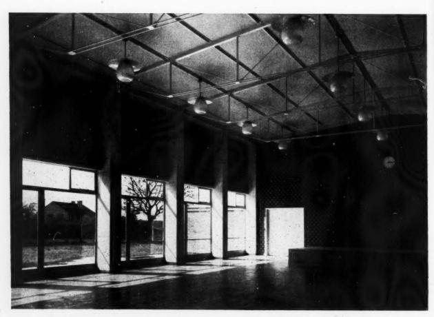
Above, the assembly hall interior. Construction is similar to that of the dining hall. A 6-deg. double-pitch lightweight welded truss has been designed to a similar pattern and using similar members to the trusses in the dining hall and classroom block. Spandrel infillings are faced with 1-in. Western
