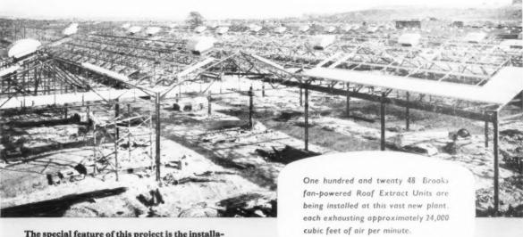
The special feature of this project is the installation of the Roof Extract Units as the steel work erection progresses.
