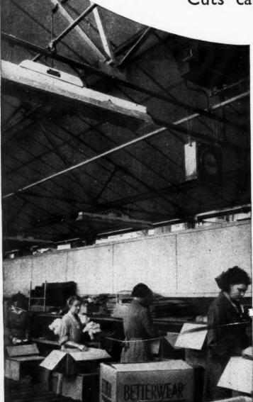
Since 1946 the roof of the Betterwear Products factory at Romford has been lined with 1/2 Lloyd Insulation Board fixed by the Lloyd Talon System. During these years, building extensions have almost doubled the floor area, yet the factory is still heated by the same plant using the same amount of coal as was needed before the expansion. Lloyd Insulation has saved heavy capital expenditure of more than £2,500 on extra heating plant and is regularly saving about £100 a week in winter fuel bills.
