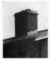
Flashing round chimney stack
