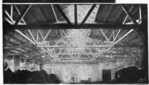
Scientifically constructed, with pre-formed bows of laminated wood.
