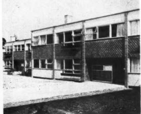
Flats at Parkleys, Ham Common, in which 4" Thermalite has been used in panel walls behind weatherhung tiling. Architect: Eric Lyons F.R.I.B.A.
