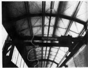
Above: the crane bay to the north of the main shop (see also viewpoints 8 and 9) has a symmetrical roof, but the same steel pre-fabricated units as in the rest of the factory have been used. To left and right at high level is the continuous glazing. Steelwork is painted grey with principal trusses and members blue grey, the remaining surfaces being white or cream.
