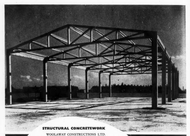
specialise in design, manufacture and erection of prestressed and reinforced concrete frames for many types of single storey building. This illustration shows the use of G.K.P. prestressed concrete trusses which span from 21 '0" to 45 '0". Early delivery and rapid erection can be arranged at economical prices. Tenders for complete buildings can also be submitted.
