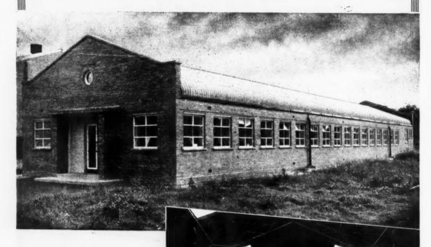
The adaptability of the Coseley Standard Steel Framed Building is shown in these illustrations. Standard Spans range from 30ft. to 75ft., with 8ft. to 20ft. height to eaves. Lean-to and canopy extensions can be supplied at standard roof slope. Lengths in multiples of 12ft. 6in. and widths in multiples of Standard spans.
