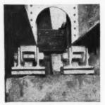
2 Rocker Bearings at one end of the Girders.
