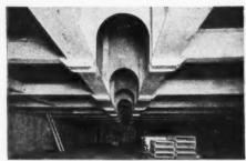
1 View of 70-ft. long Twin Welded Girders underneath Arrested Landing Deck.
