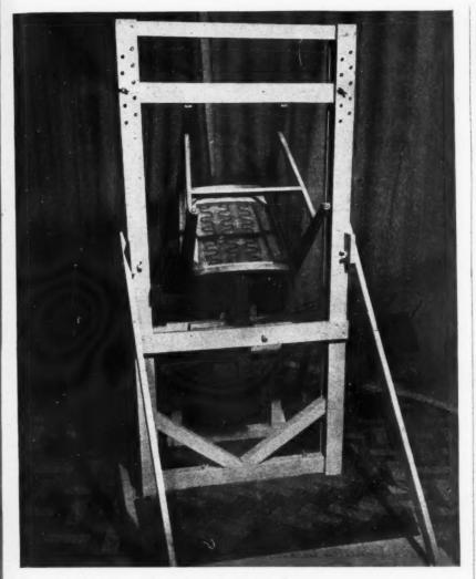
Fig. 4, a standard test for establishing the strength of the joints in a chair.
