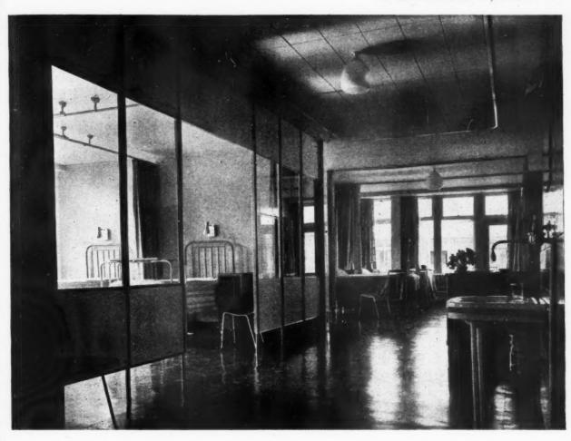
Above and below: interiors of a typical ward. Acoustic tiles are provided over the corridor area; the cork or semastic floor tiles are finished with a plastic sealer. Radiators and piping are exposed at the perimeter of the ward under the windows. Each patient has a reading light under his personal control, and the general lighting is from large opal fittings close to the ceiling.
