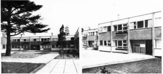
Flats at Parkleys, Ham Common, in which 4" Thermalite has been used in panel walls behind weatherhung tiling. Architect: Eric Lyons F.R.I.B.A.
