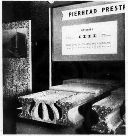
Top: rubbed rubber sheeting for patterning precast concrete slabs. See item (right) on British Rubber Development Board. Above: Picrhcad Ltd.'s prestressed concrete beams with lightweight concrete pot infilling. See page 737.
