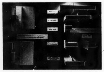
Above: detail from Williams & Williams Ltd.'s stand, showing typical aluminium extrusions used on Wallspan curtain walling. Below: external view of part of Williams & Williams Ltd.'s stand, showing Wallspan in use. (See page 741.)
