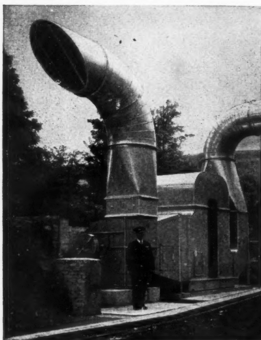
The illustration shows one of four large fume extraction plants entirely constructed of T I Aluminium in a modern factory in South Wales.
