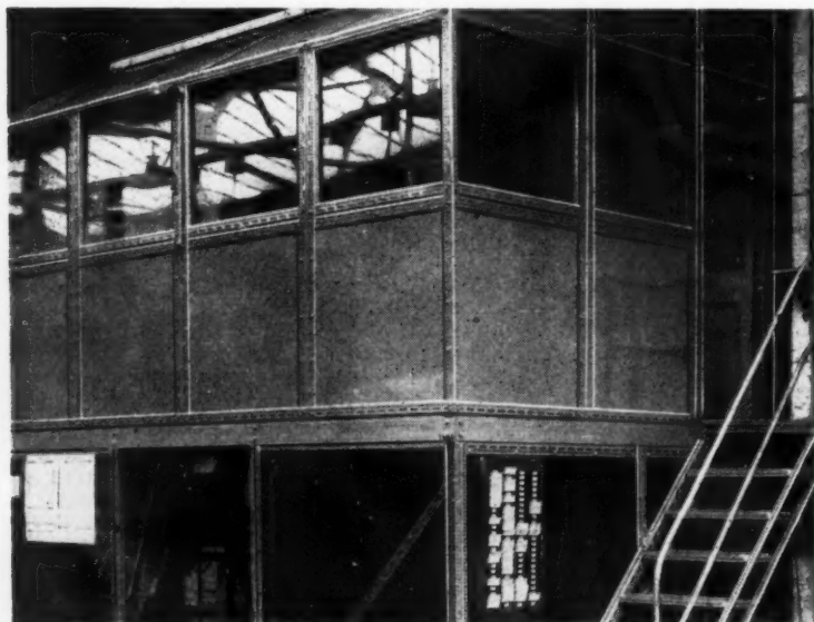
Machine Shop Engineer's office quickly built. Thomas Allan & Sons Ltd. of Thornaby designed this office with tool store underneath to be built with conventional materials. They used Dexion instead when they found it was quicker and cost less. In jobs of this sort, Dexion invariably supersedes old-fashioned materials and methods.
