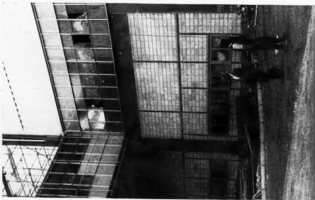
The concrete block wall round the base of the turbine hall, showing the effect of the 9\frac{3}{4} -in. module and 13-ft. steelwork grid. The concrete blocks are 9\frac{3}{4} in. high by 1 ft. 7\frac{1}{2} in. long by 10 in. thick and were pre-cast on site.
