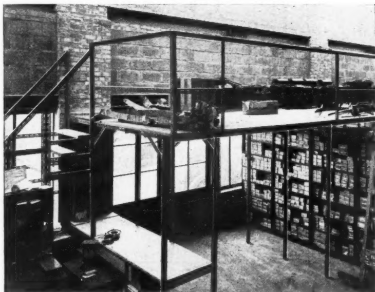
Service Depot builds storage platform. Iron Bridge Service Depot Ltd. of Southall, Middlesex, built this overhead storage platform to carry 20 tons of motor-car parts. It effects a big saving in space, and the supports also serve as dividers for storage bins. Storage structures of Dexion can make full use of any existing space; and they have the great advantage of ensuring easy adaptability to changing needs.
