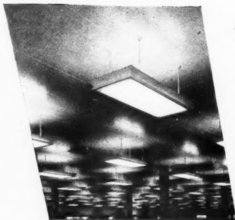
ASBESTOLUX ceiling panels screwed to suspended tee sections at the Lewisham branch of British Home Stores.
