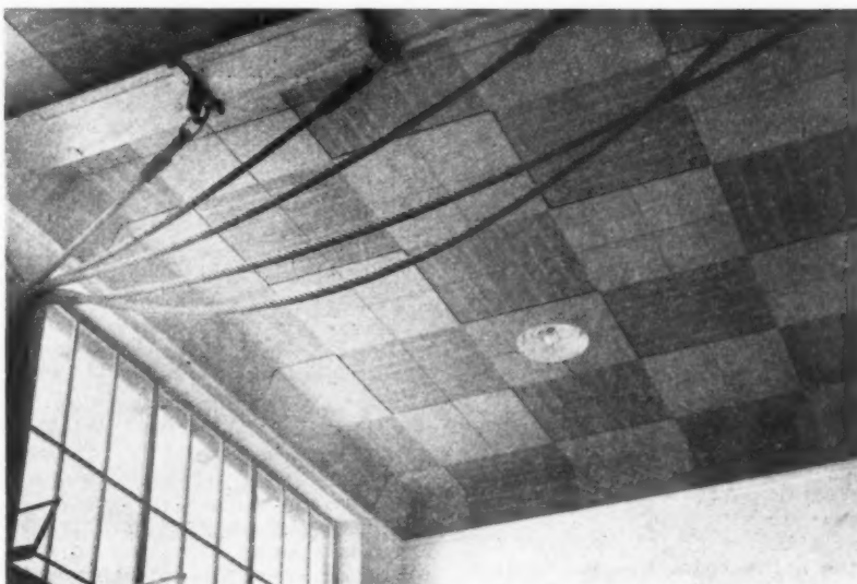
Fig.2. Slotted and perforated tile ceiling in a gymnasium.
