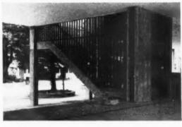
Left, Fig. 9, secondary staircase on block C landing on covered play space. Note service duct built into the column on the right. Below, Fig. 10, detail of junction between monitor roof lights over changing rooms and clerestory of gymnasium.
