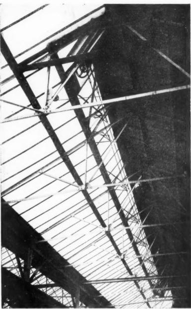
The illustration shows One set of Electrically operated Twin Tension Rod Gear with Counter-Balance Unit operating one continuous opening light, 74' 0" long × 5' 0" deep. Note the Spiral Balance Wheel fitted at the end sprocket.
