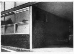
Fig. 8, finishes adjoining covered play space in block C. Left, "stable yard tile" plinth; right, glazed limegreen frost-proofed tiles.
