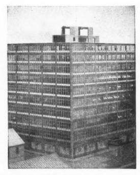
Wallspan is going up all over the world! The recently completed Commonwealth Building in Ottawa (Architects: Abra and Balharrie) has Wallspan on all four elevations. An interesting feature is that the louvred spandrels are backed with removable insulating boards which in hot weather are replaced with panels incorporating extractor fans.
