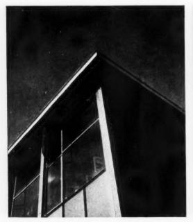
Left, Fig. 4: detail of troughed eaves of the Howard School and composite window construction. In this school, the last of the programme, certain gable walls were built in facing brickwork, in the absence of an alternative cladding, to assist in articulation of the building. Right, Fig. 5: corridor in the main administration block of the
