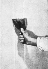
Final coat of GYPROC Joint Filler applied with a 5" wide rigid joint filling knife.
