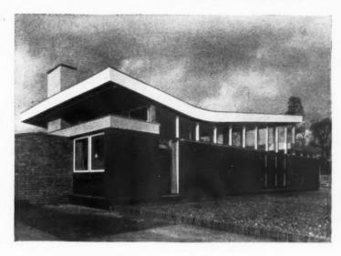
east. The external walls here as elsewhere in the building are 10½-in. cavity construction of two skins of 4½-in. expanded clay blocks. The external finish is a dark grey cement spatter. Opening windows are painted white, and the casement doors black. The clerestory window mullions support the roof.
