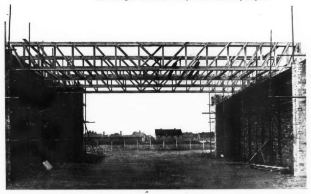
\*Aerolite' -- glued roof truss for the assembly hall of a school at Marsk-on-Sea. Architect: J. H. Napper, M.A., F.R.I.B.A. Structural Engineer: D. W. Cooper, B.Sc.
