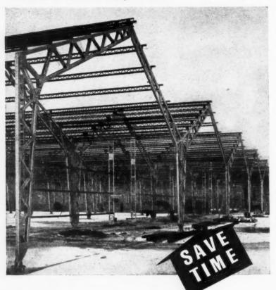
The Metsec technique for portal frame buildings is responsible for a number of important advantages, all of which contribute to the basic characteristic of the system—SAVING COST BY THE SAVING OF TIME AND LABOUR
