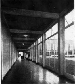
Howard School, looking towards the entrance hall and assembly hall. The lattice beams are cased in fibrous plaster (2-storey block) to provide necessary fire protection. The stanchion casings and window cornice are also in fibrous plaster. The ceiling is in 1-in. fine woodwool tile screwed to battens.
