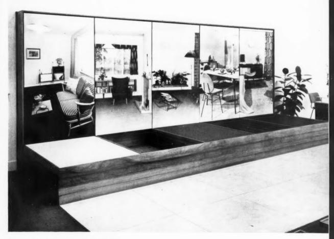
The object of this case is to display carpets in approximately the same plane in which they will be seen in use while avoiding the exhausting practice of lifting up each piece and throwing it back over a roll. The three uppermost surfaces of the case are fixed: beneath each are five movable trays which are suspended on sliding door gear and which can be slid into view in one or other of the two wells.
