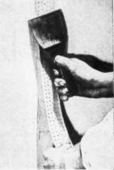
Embed GYPROC Perforated Joint Tape whilst GYPROC Joint Filler is still plastic.
