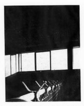
Left, Fig. 6: the Howard School; detail of suspended woodwool tile ceiling, showing the use of fibrous plaster margin cornice to overcome the need for cutting. The ceiling pattern is offset from the structural grid. Right,
