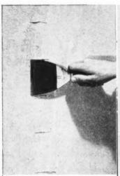
Apply a thin layer of GYPROC Joint Filler into recess with a 4" wide flexible joint filling knife.
