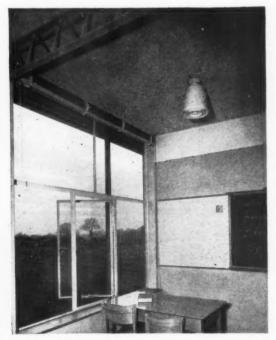
Fig. 7: detail of junction of partition, ceiling and window in the Howard School. The ceiling is of perforated plasterboard with glass fibre backing. Note fibrous plaster casing to Presweld beam over partition.
