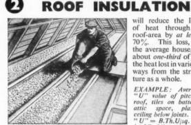
will reduce the loss of heat through a roof-area by at least 70%. This loss, in the average house, is about one-third of all the heat lost in various ways from the structure as a whole.
