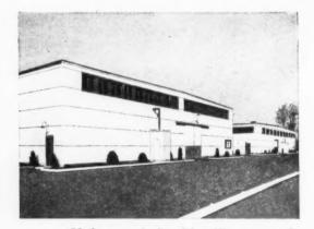
Modern methods of handling materials have started a trend towards singlestorey warehouse buildings. Timber construction fulfils all requirements for structures of this type at reasonable cost.
