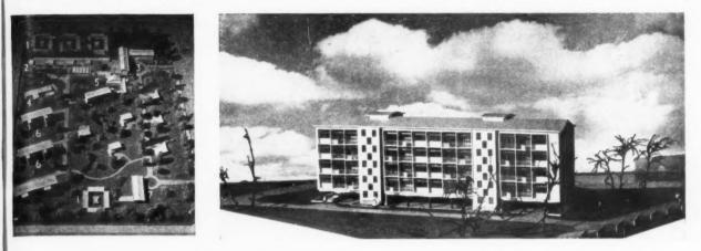
16 flats, open on the ground floor, except for stores, entrance halls, lifts and staircases. The flats will have a r.c. frame, and walls of light weight concrete blocks, finished externally with rendering, glass mosaic or tiles. The roof will be covered with ribbed alu-
