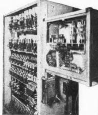
The main lift controller and electronic control equipment, which can be sited in any convenrent position. Right: Factual speed/time curves for this electronically controlled lift Below: Drum mechanism, embodying cams and followers of the control gear, photographed across the lift shaft.
