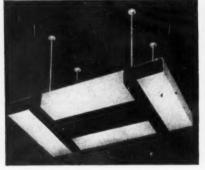
op, Fig. 11. Philips' "Amersham" gearless fluorescent fitting. Above left, Fig. 12. Light fitting built up from Atlas "Domino" fluorescent units,
