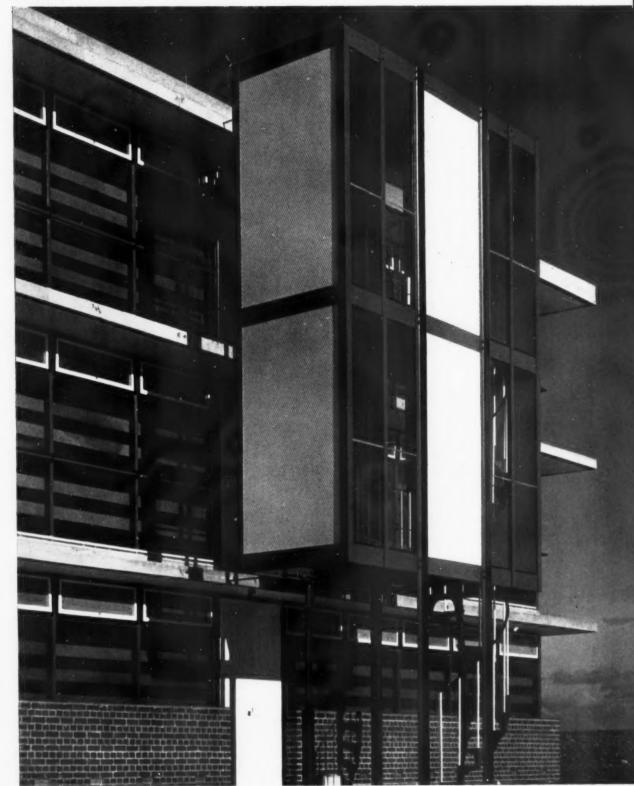
The enclosure protects hoist, stairs and landing : its form was dictated by the need to separate the enclosure from the warehouse building so that the former cannot act as a flue in case of fire. Solid panels of steel plate serve as bracing in place of the more usual diagonal struts or ties and are designed to withstand swinging or leaning sacks. The structural metalwork is shot-blasted, chromate-sprayed and painted four coats.
