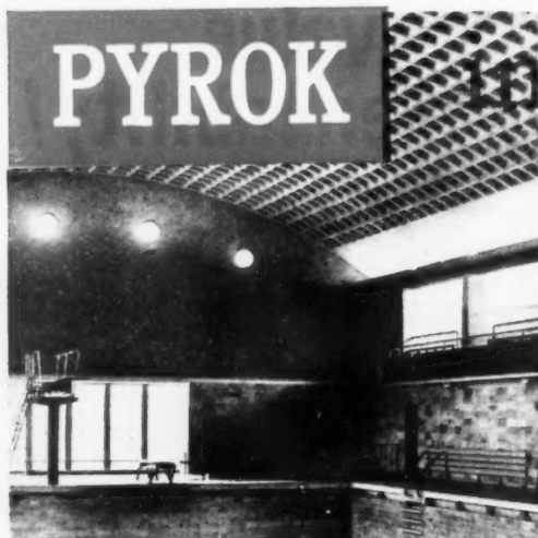
The illustrations from Hameln, Essen, Cologne and Bochum in Germany show the use of Pyrok as an anti-condensation and acoustic treatment to ceilings
