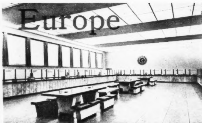
The illustrations from Hameln, Essen, Cologne and Bochum in Germany show the use of Pyrok as an anti-condensation and acoustic treatment to ceilings
