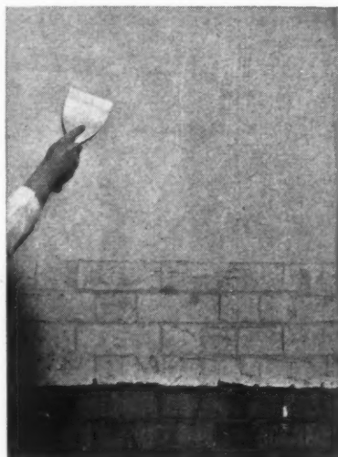
1 Fillex being applied over brickwork
