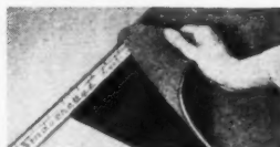
Carpet is hooked on to "Smoothedge" plywood strips; edges are tucked over and tightly sealed between strips and wall.
