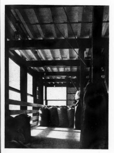
A view typical of the three floors of the processing block. The processing of seeds is primarily a vertical operation necessitating numerous perforations in the floors and in consequence the architects decided on a softwood boarded floor construction with soffits exposed on certain floors. The softwood stacking rails running around the perimeter of the rooms are fixed back to the structural steelwork and intermediate glazing mullions.
