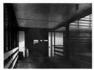
The artificial drying room is located on the top floor of the processing block. The apparatus on the right comprises a gas heater, fan and ducting. The seed drying area on the left is warmed by air passing through floor ducts and grilles served from a gas heated plenum chamber. After drying, the seed is poured through chutes to the floors below for further processing. Colour: apparatus—yellow: ceiling and bottom hung vents—white; steelwork—crimson; sliding door—dark blue.
