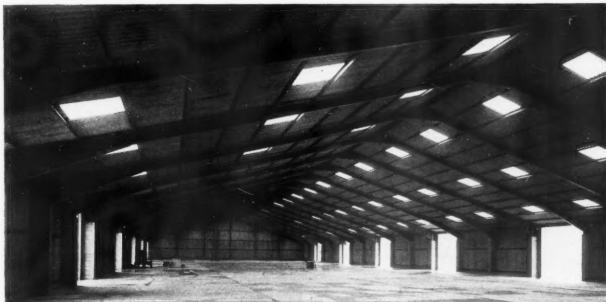
Warehouse Length 300 ft. Span 101 ft. - 6 ins. Pitch 17° Architects: Fowler Grove & Haggard Southampton.
