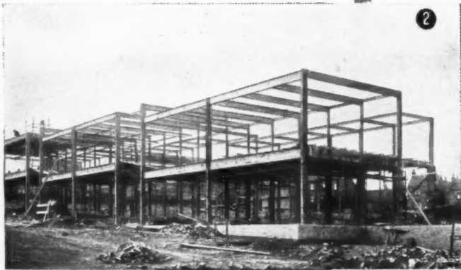
1 New factory building for Messrs. William Cooke & Sons of Rotherham. 300 ft. x 120 ft. span.
