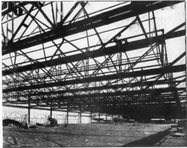
1 New factory building for Messrs. William Cooke & Sons of Rotherham. 300 ft. x 120 ft. span.
