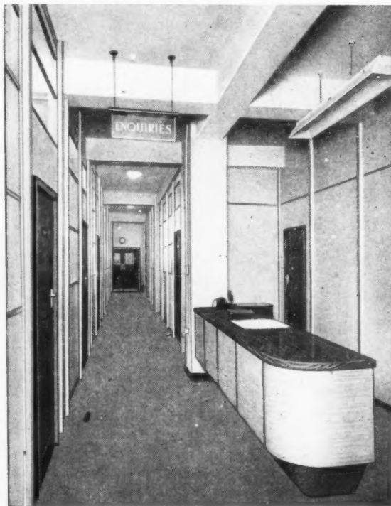
Demountable partitioning by Compactom Ltd., in the City Offices of The Shell Petroleum Co. Ltd.
