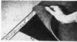
Carpet is hooked on to "Smoothedge" plywood strips; edges are tucked over and tightly sealed between strips and wall.
