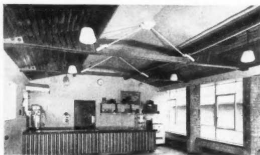
The staff canteen in the centre of the administrative building. The brick pillars and external walls up to sill height are of concrete bricks; the walls being of 11-in. cavity brick construction. The floor is finished with 4 ft. by 2 ft. 7 in. in situ granolithic paving, divided by ebonite strips. The door in the far wall leads from the kitchen to the service counter.
