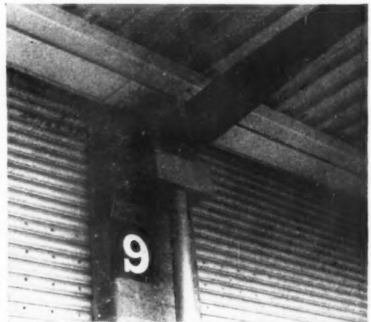
Viewpoint 9: detail of rain-water head under canopy. This enables the canopy to be drained and also allows the rain-water pipe from the clerestory to clear the cantilever.
