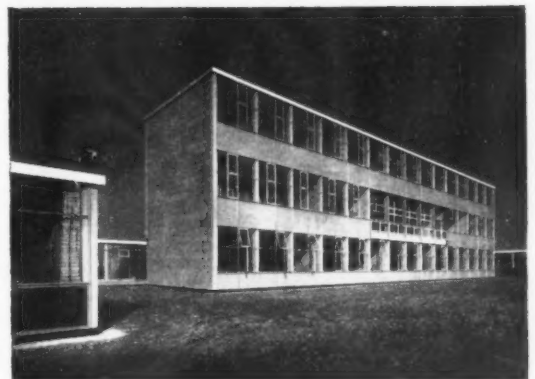
Top, Fig. 1: detail of cladding of three-storey block at the Heathcote School, Stevenage, showing vertical cedar weatherboarding included within the window construction. The curtain does not extend to ground floor level. Concrete cladding is used in two colours to articulate the form of the blocks. Above, Fig. 2: detail of cladding of three-storey classroom block at the Bennetts End School, Hemel Hempstead. Here the window construction has been developed into a full curtain wall reaching from eaves to ground. The panels are wired cast glass with Asbestolux panels behind, which are removable for painting and cleaning. The library on the first floor receives a different elevational treatment.
