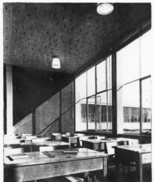
Two alternative ceiling treatments at the Heathcote School, Stevenage. Left, Fig. 6: the use of perforated plasterboard (note also the built-in blackout blinds at window head); above, Fig. 7: the use of perforated fibrous plaster panels spanning between floor beams.
